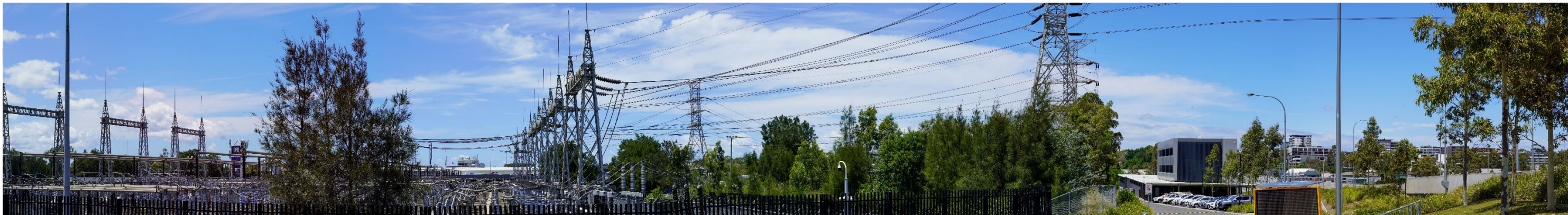
Figure 0-1 Viewpoint 1: Existing view
