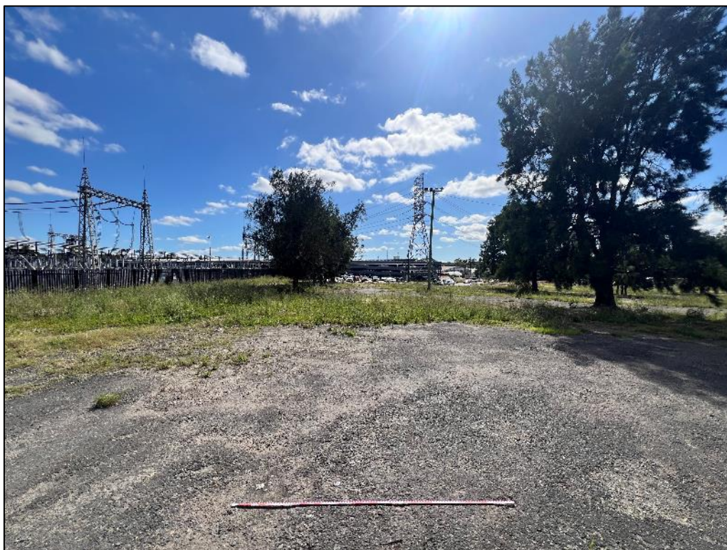
Plate 7: Looking north towards the DFO facility and STSS.
