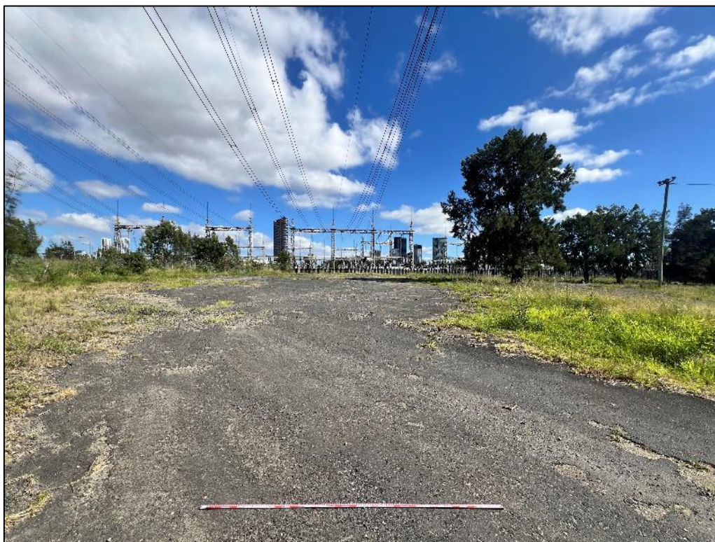
Plate 6: Looking west towards the existing STSS.
