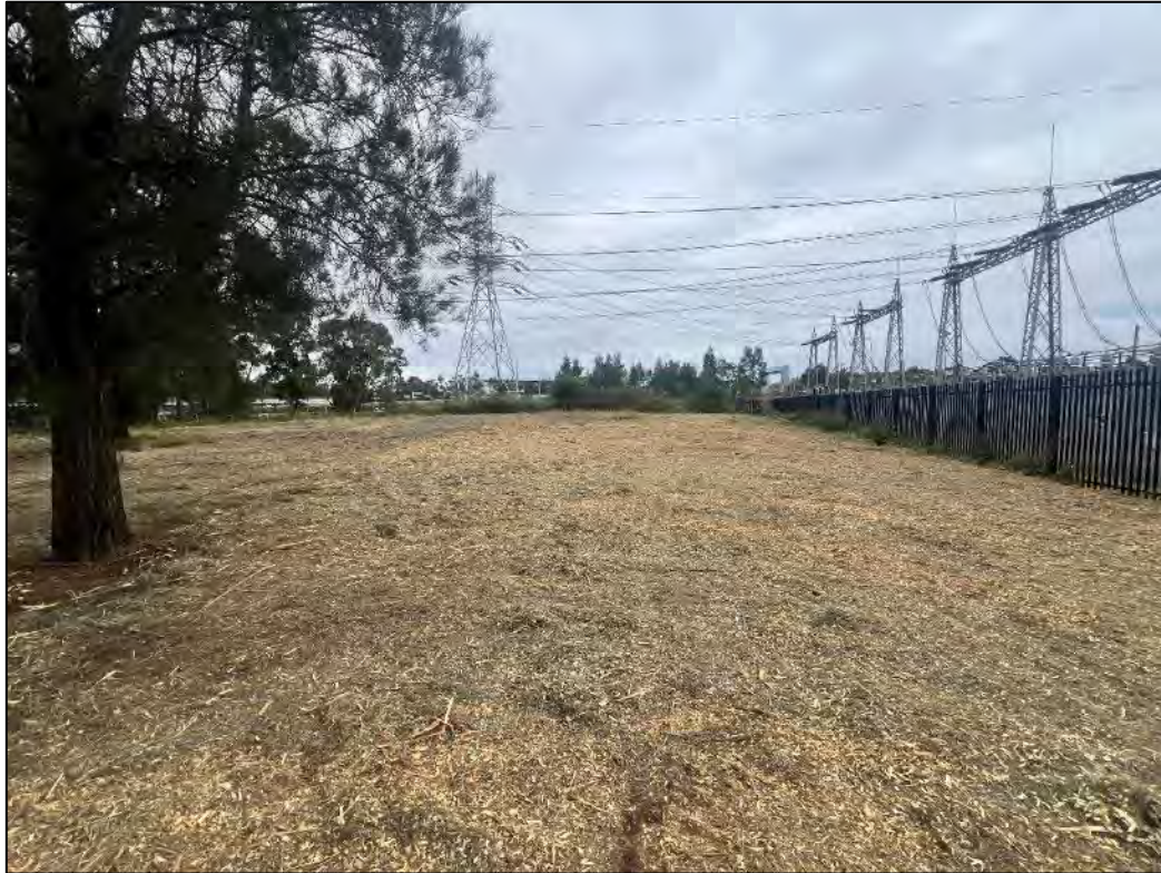
Plate 10: View showing further vegetation clearance along the northern boundary with the Zone Substation
