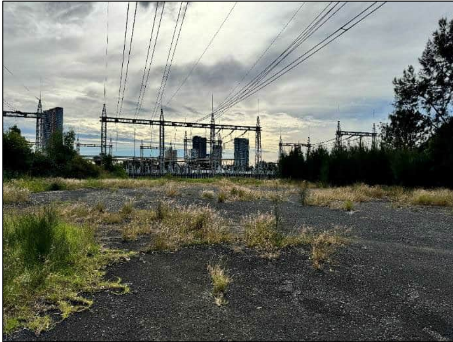
Above: View north from centre of the Subject Site
