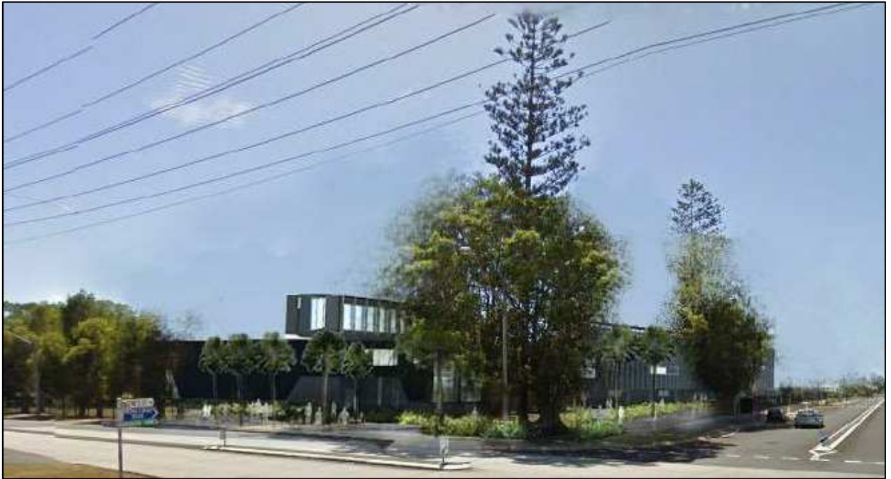
Figure 17: View of BCHS from the corner of Swift and Cherry Streets (Source: Applicant's EIS)
