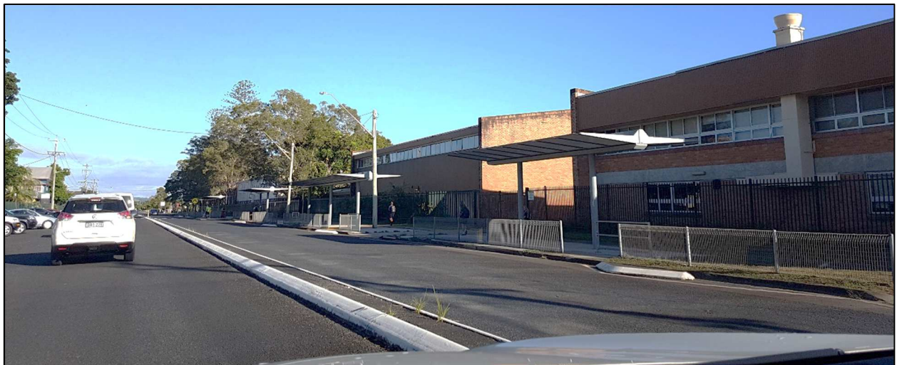
Figure 6: View of BHS from Swift Street (Source: DPE)
