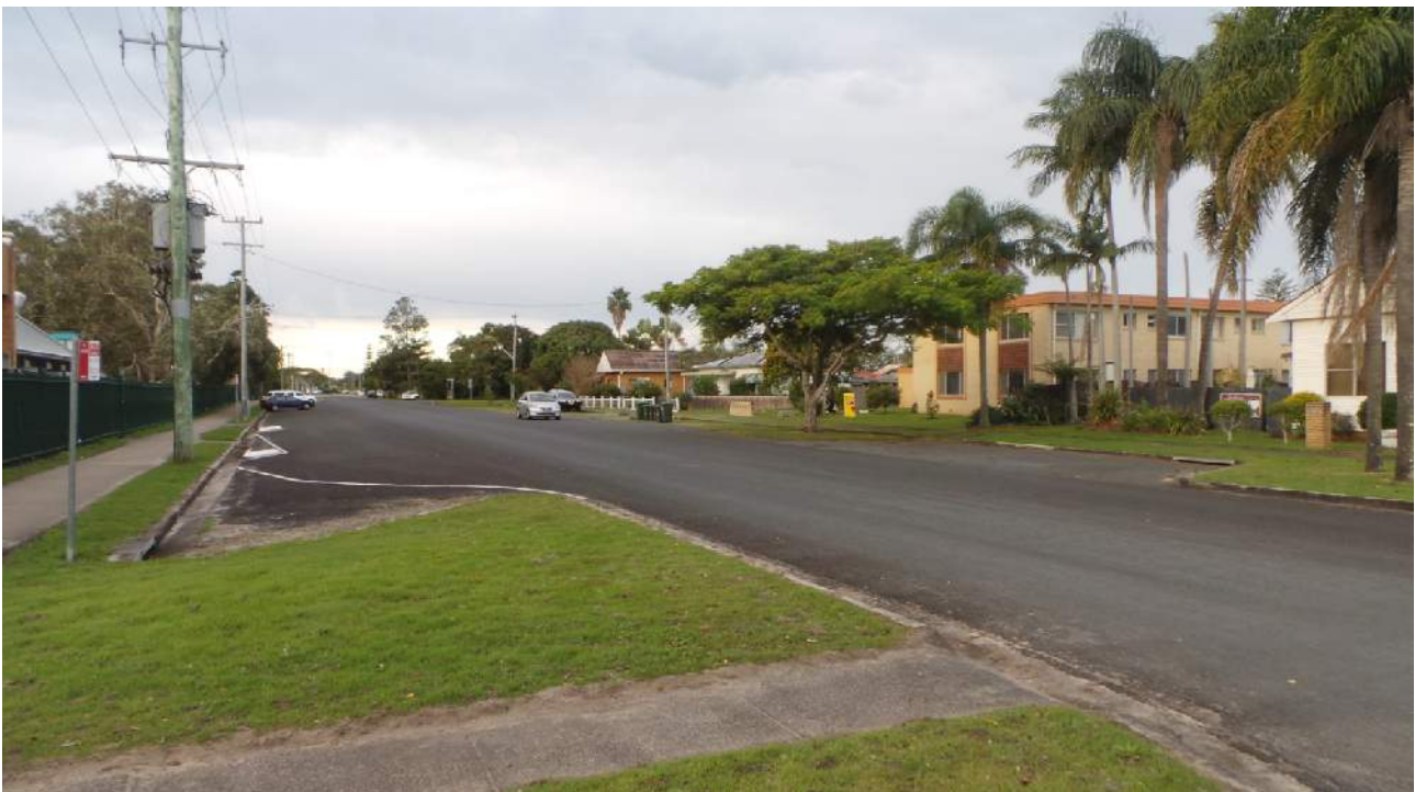
Martin Street at Swift Street Intersection, view to the north
