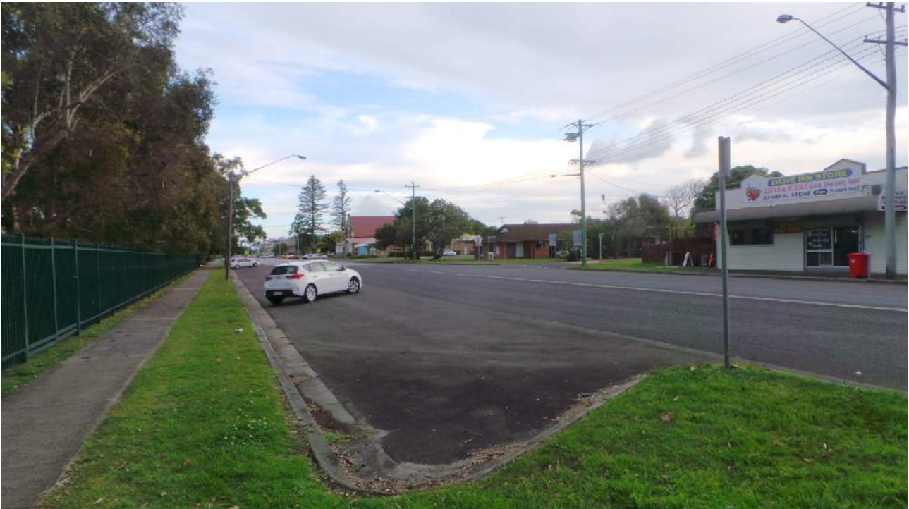
Cherry Street at Burnet Street Intersection, view to the south
