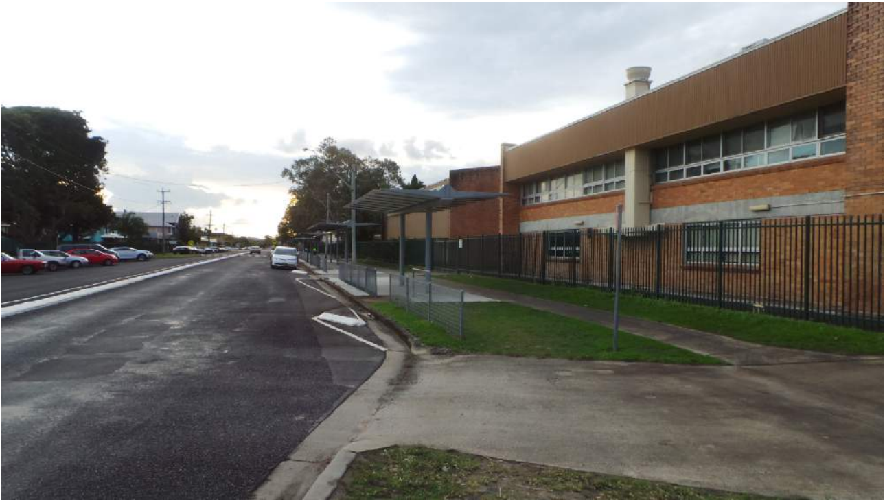
Swift Street at Martin Street Intersection, view to the west
