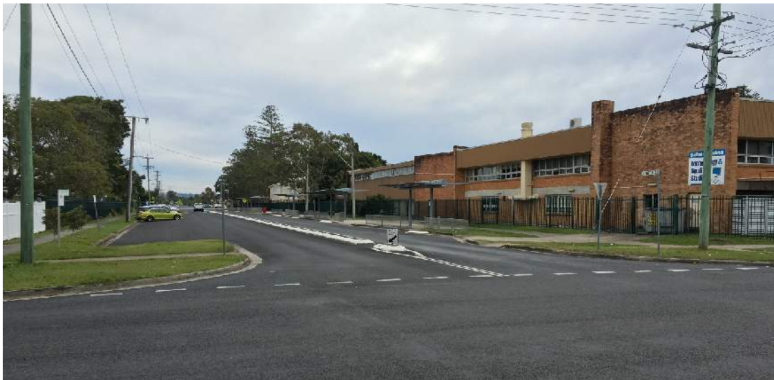
Swift Street at Martin Street Intersection view to the west
