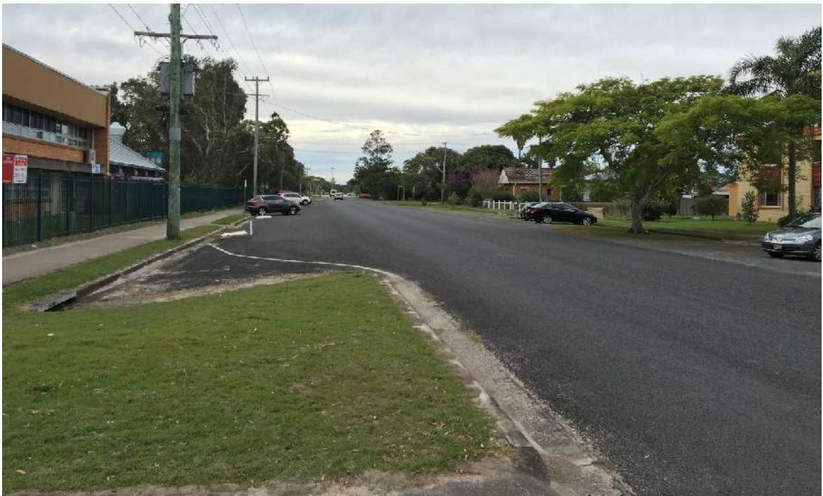
Martin Street at Swift Street Intersection view to the north
