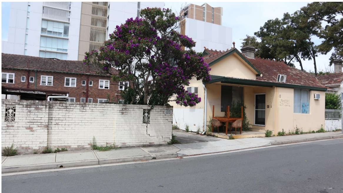
Figure 32: Rear access to No.20, No.22 and No.24 Railway Parade and chief elevation of No.2 Burleigh Street.
