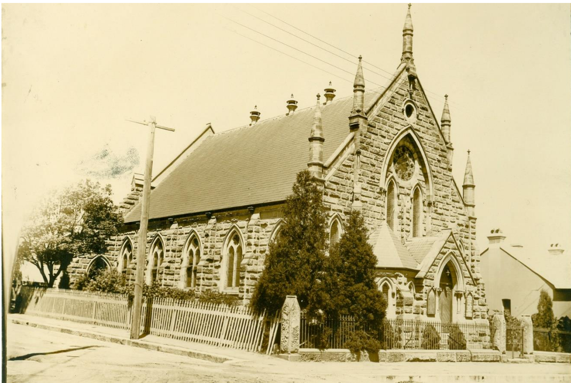
Figure 20. Methodist Church c.1920, adjacent to subject site (Source: Burwood Council)
