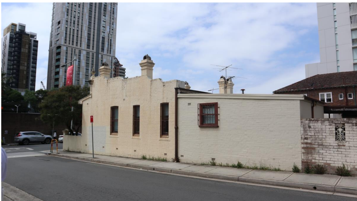
Figure 30: Side elevation of No.24 Railway Parade, from Burleigh Street
