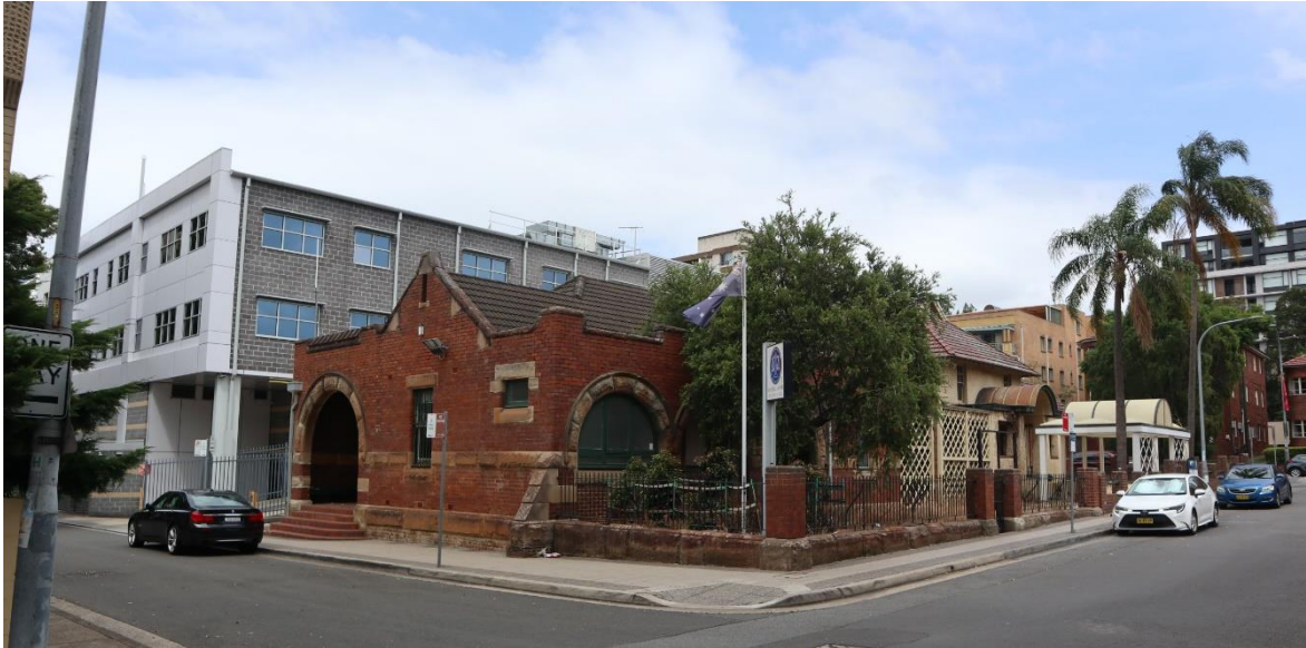
Figure 39: Former Police Station and Courthouse on corner of Burleigh Street and Elizabeth Street.
