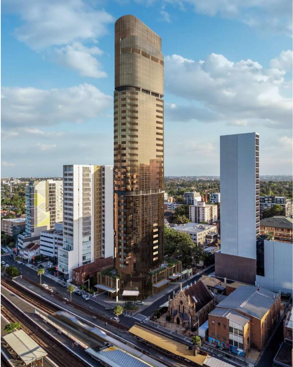
Figure 45: Proposed Perspective viewed from above Burwood Railway Station onto the subject site.
