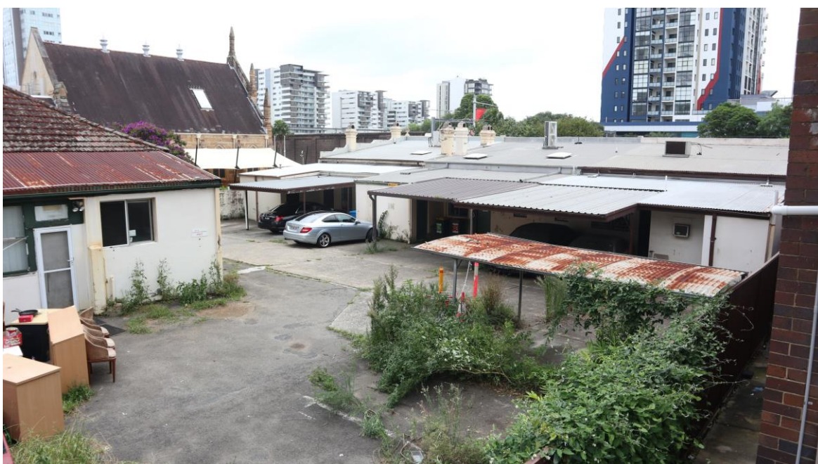
Figure 31: Rear elevations of No.20, No.22 and No.24 Railway Parade and No.2 Burleigh Street.
