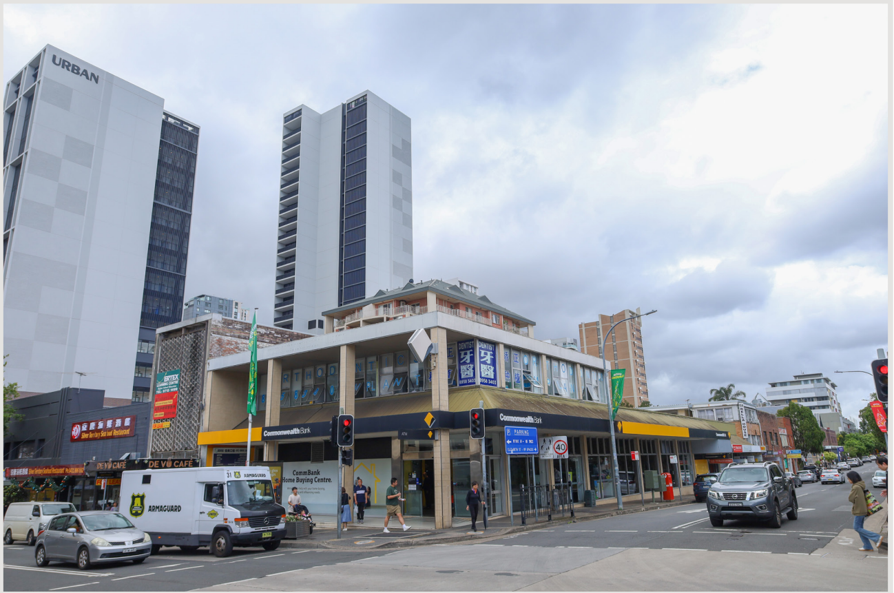
Existing site photo - Burwood Road.
