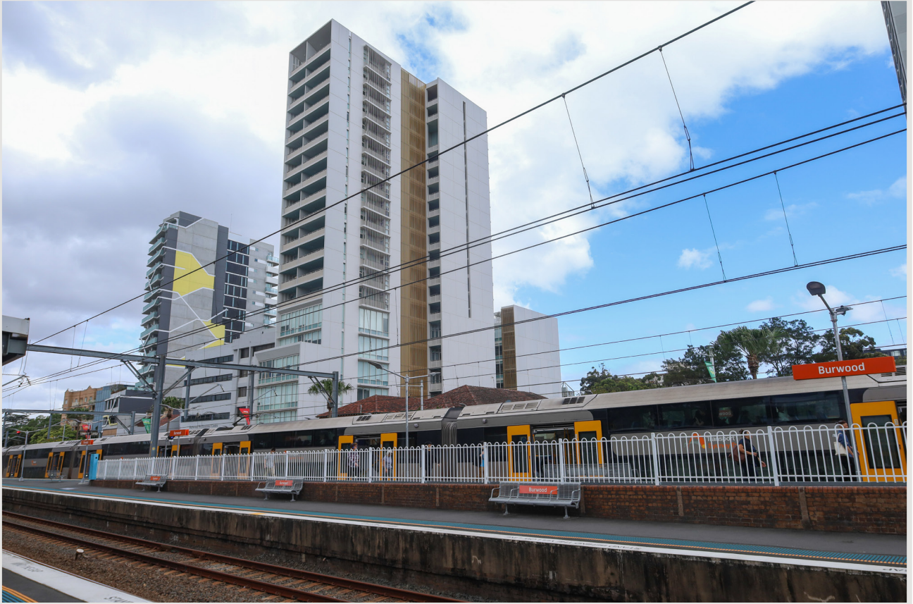
Existing site photo - Burwood Station
