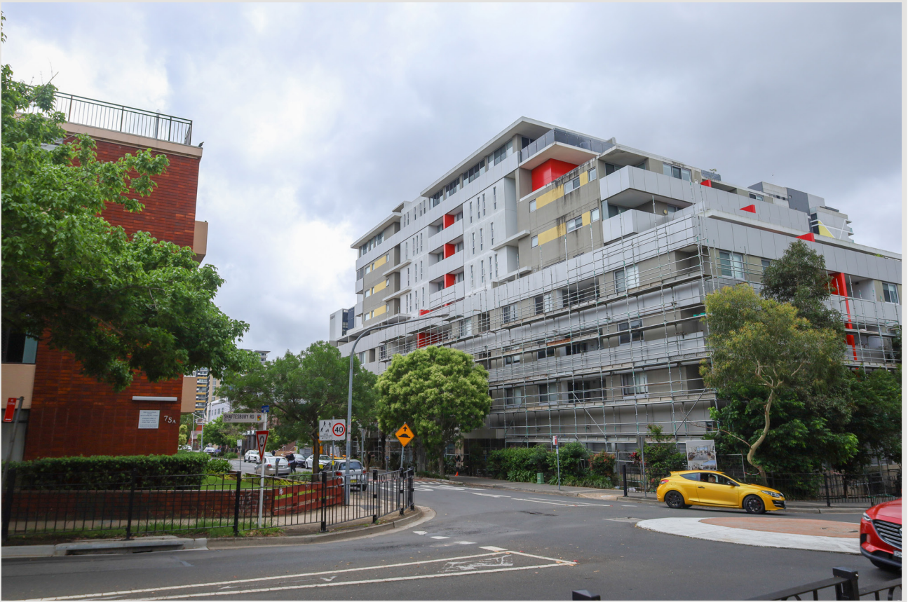
Existing site photo - Shaftesbury Rd
