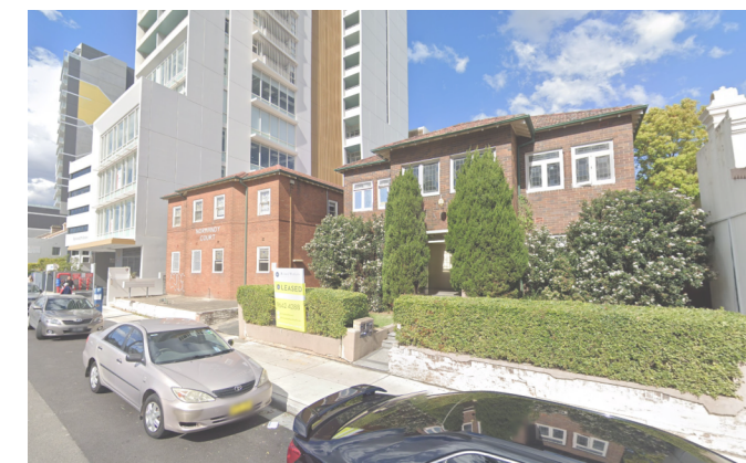
Residential flat buildings no. 18-18A Railway Pde
