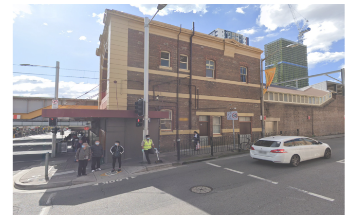
Item 2 - Burwood Train Station
