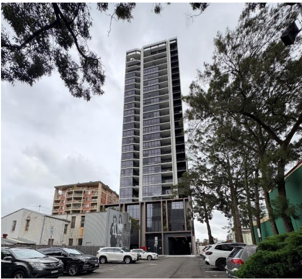
Figure 19 No. 7-9 Burleigh Street, viewed from council carpark.
