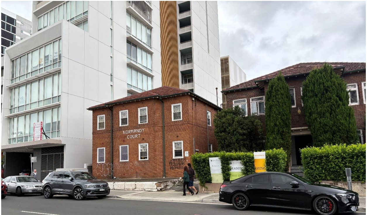
Figure 13 Development immediately east of the subject site.
