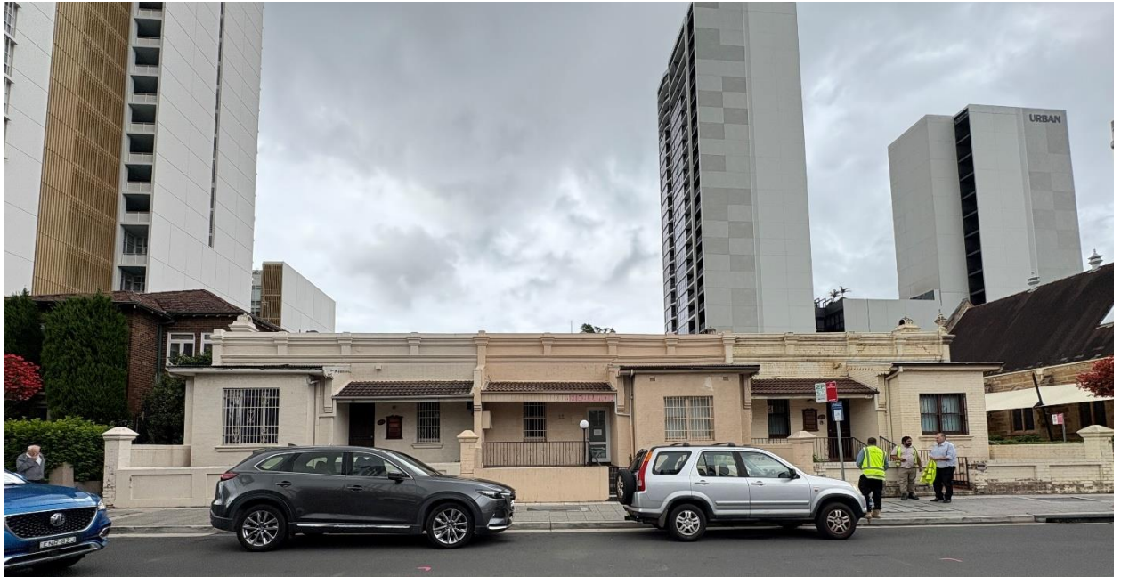
Figure 3 The subject site, as viewed from Railway Parade.
