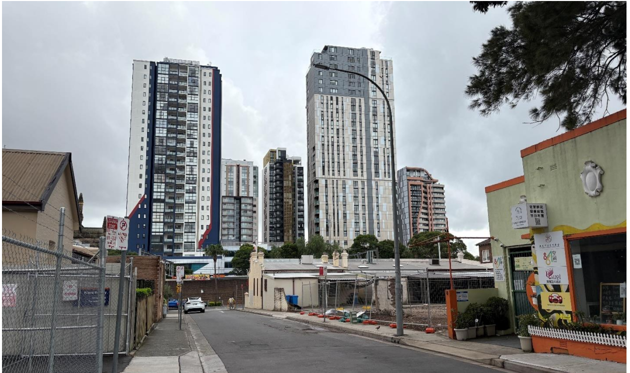
Figure 6 Mixed use development to the north of the railway, as viewed from Burleigh Street.
