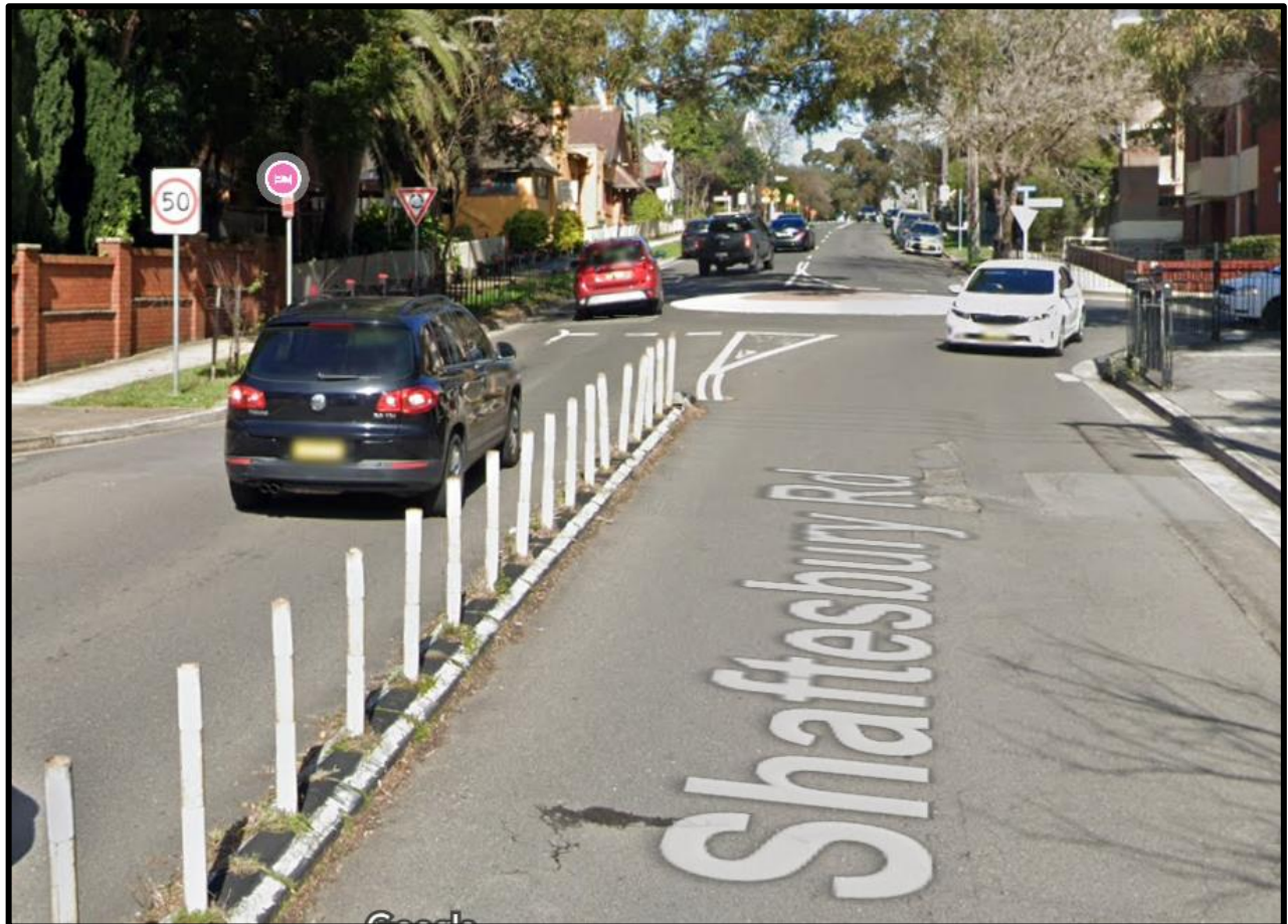
Figure13: Street View of Shaftesbury Road Looking South (Source: https://www.google.com/maps )
