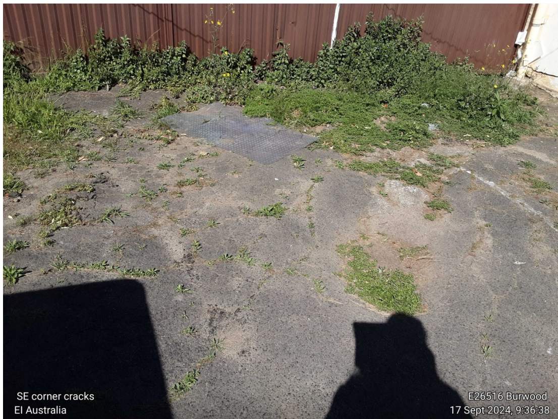
Photograph 6: The surface of the carpark.
