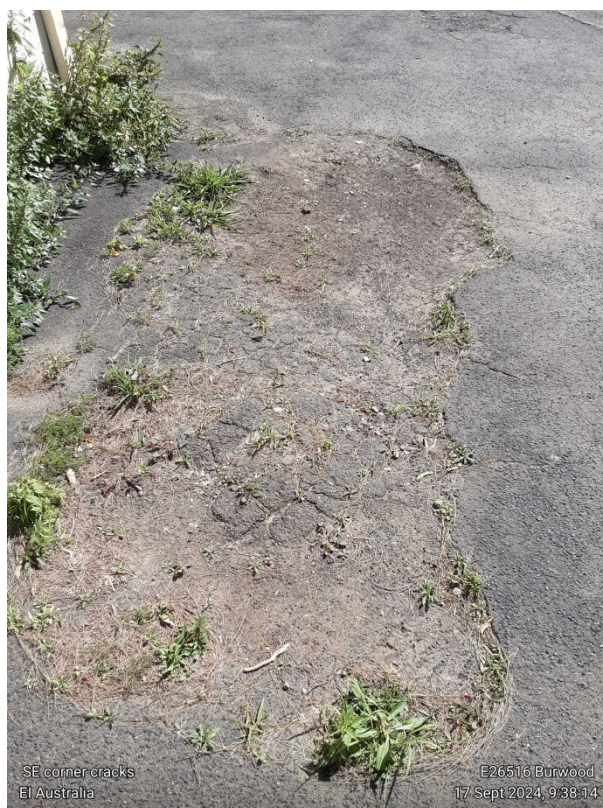
Photograph 7: The surface of the carpark
