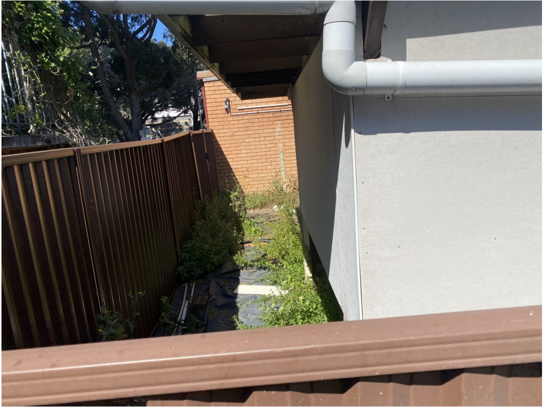
Photograph 11: Backyard of 4 Burleigh Street, facing south.
