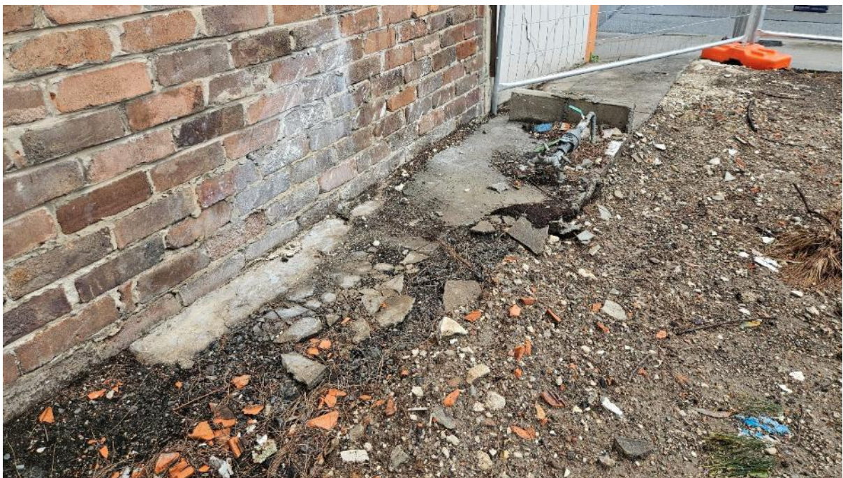
Plate 12. Foundations and exterior wall of the neighbouring 6 Burleigh Street. (Source: Heritage Now 2025)
