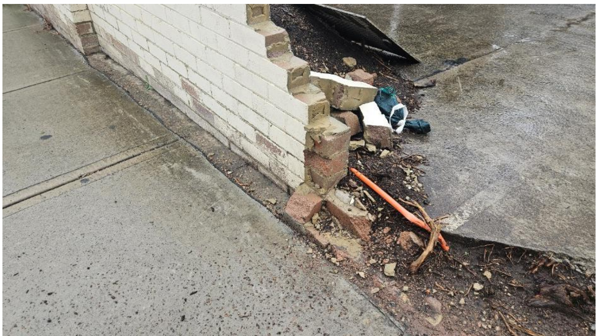
Plate 6. A service line, tree roots, and a brick wall foundation visible underneath the concrete driveway. (Source: Heritage Now 2025)
