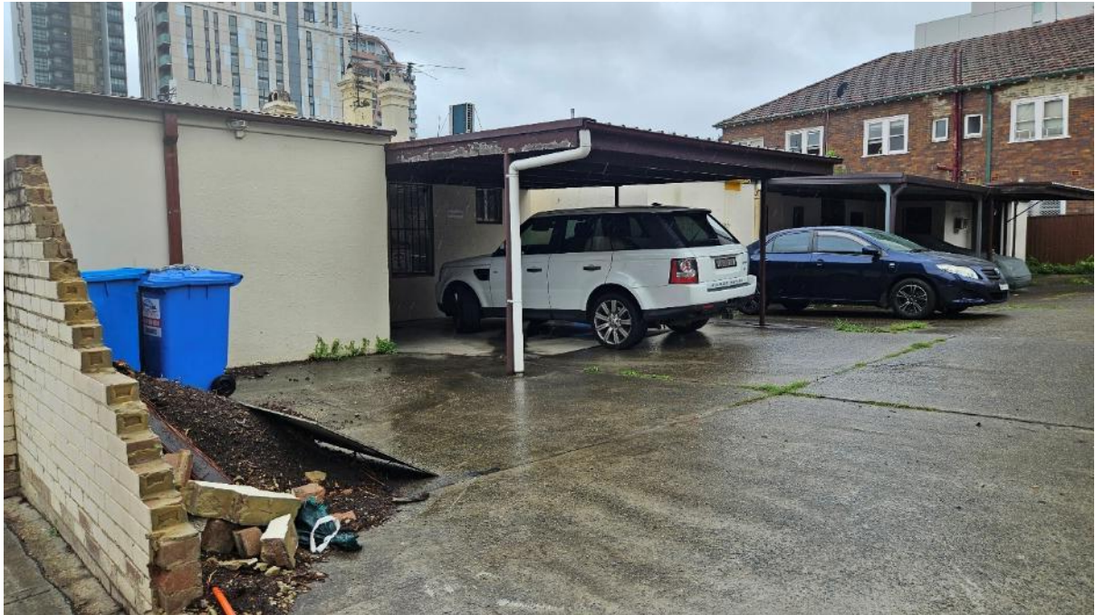
Plate 1. Buildings and concreted areas within the Project Area. (Source: Heritage Now 2025)
