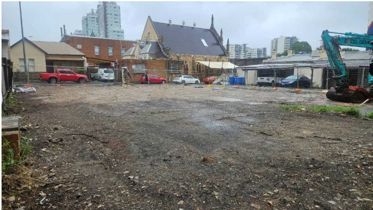
Plate 7. The southern portion of the Project Area where the Burleigh Street buildings have been demolished. (Source: Heritage Now 2025)
