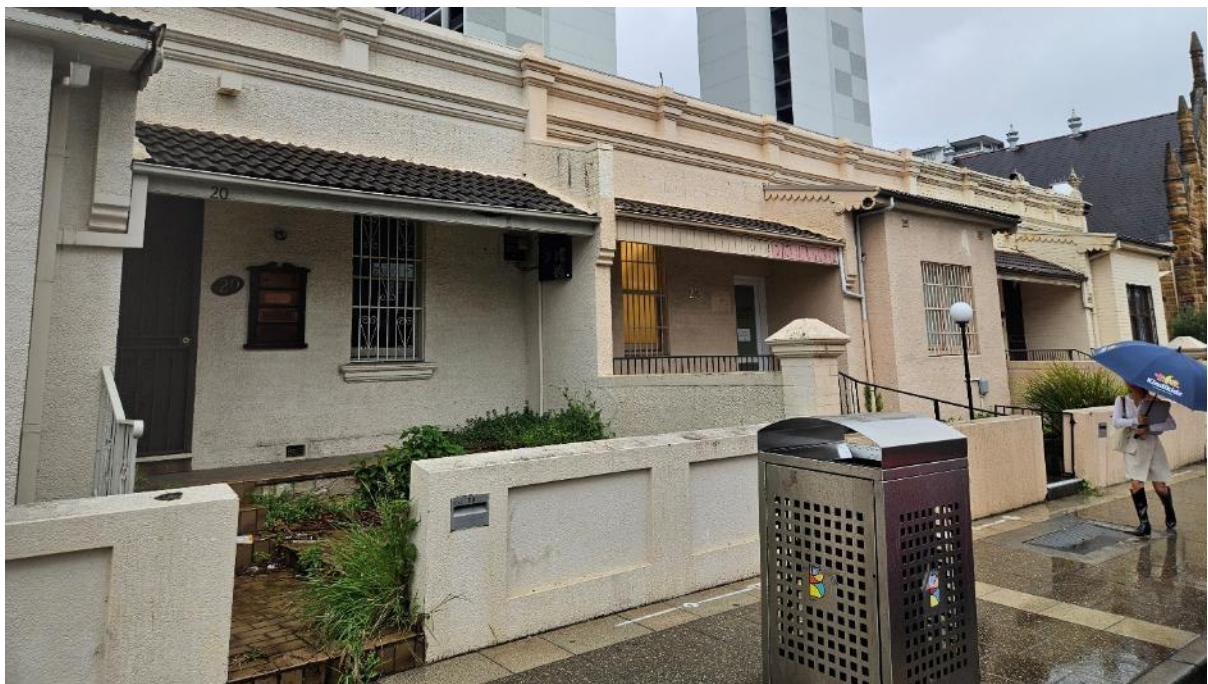
Plate 3. The front of the buildings have been somewhat built up off the ground. (Source: Heritage Now 2025)
