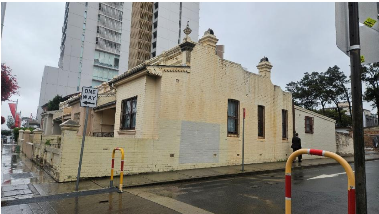
Plate 2. The remaining buildings, showing the slope towards Railway Parade. (Source: Heritage Now 2025)
