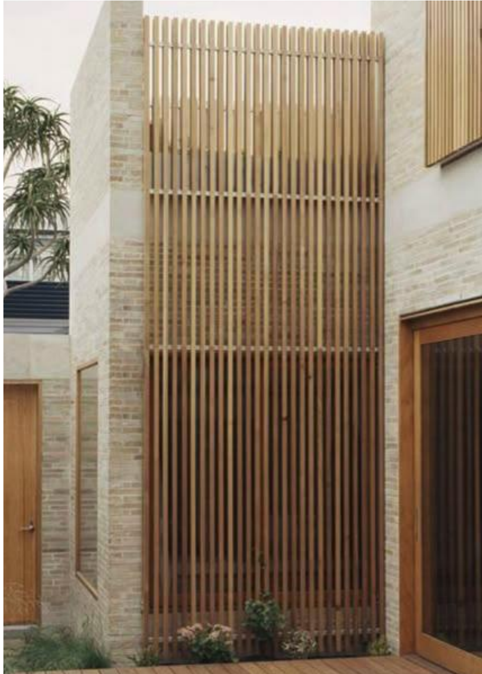
SC 01 VERTICAL TIMBER-LOOK ALUMINIUM SCREEN
