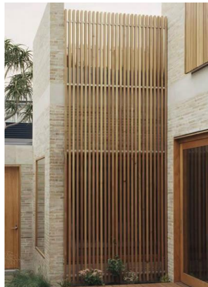
SC 01 VERTICAL TIMBER-LOOK ALUMINIUM SCREEN
