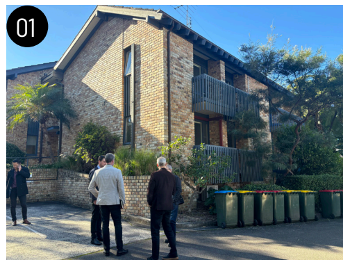
EXISTING AGED CARE FACILITY
