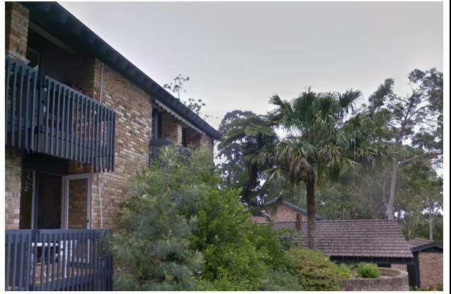
Existing aged care facility looking from west from Main Drive
