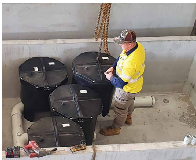
FIGURE 2 AtlanFilter install
