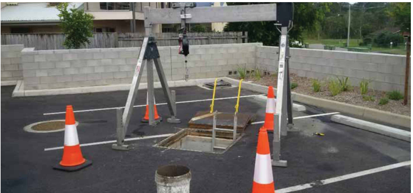
FIGURE 4 AtlanFilter install set-up
