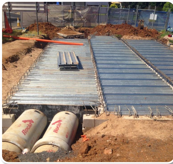
Detention Tank during construction
