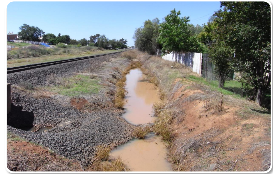
View along the Rail Corridor swale with the hospital to the left of the picture
