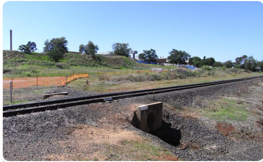
View from Rail Corridor looking South East towards the hospital
