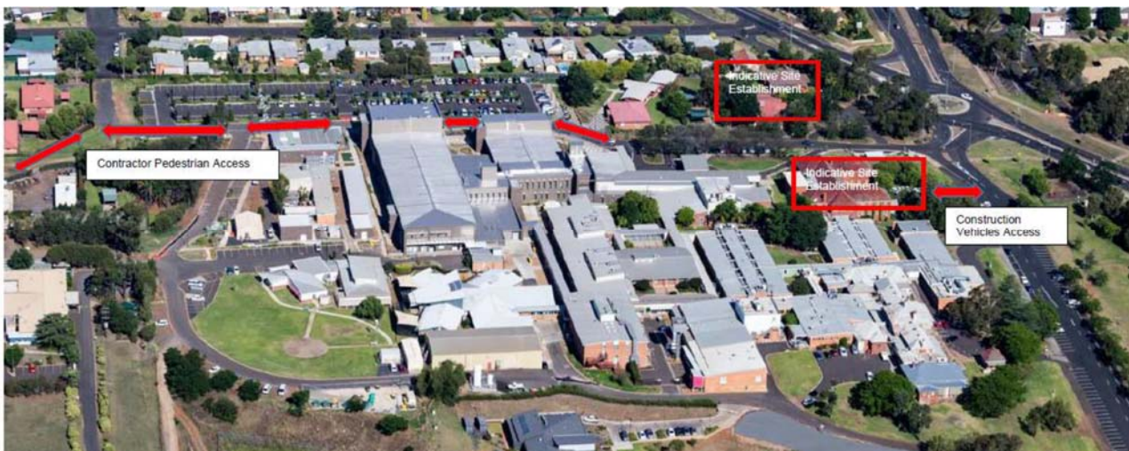
Figure 4 – Indicative Contractor pedestrian access (from north)
