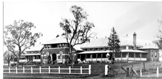
Figure 26 Photo showing the 1913 wing completed. The gable to the left is now the west gable of the partly demolished 1868 building. The transverse gable now facing towards the 1913 wing is the temporary means of addressing the exposed roof space. Incidentally, this is almost the view that could potentially be recovered if the 1966 building was removed and the verandahs reinstated (see below) - Macquarie Regional Library Local History
