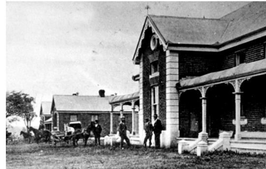
Figure 17 The two buildings formed a streetscape that had a high degree of unity from 1887 to 1907. Macquarie Regional Library Local History
