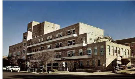
Figure 51 Cowra Hospital was originally designed for Dubbo by Cobden Parkes 1947-1950. 46
