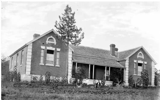
Figure 9 Photograph of hospital shortly after it was built, dated 1870-75. The shadow of the kitchen can be seen at the rear. SLNSW PXA 4999 Holtermann Collection - Home and Away – 40091
