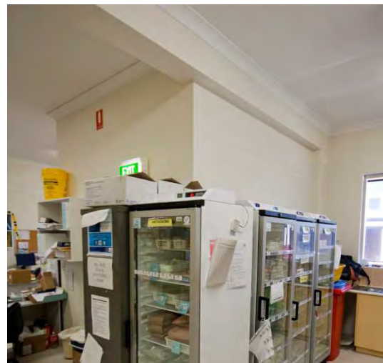
Figure 38 A large section of the original internal wall has been removed to open into an adjacent space, and a lightweight partition encloses a space – Adaptive Architects Pty Ltd 2014
