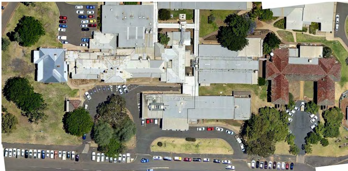
Figure 3 Aerial photo of the Myall Street frontage taken in November 2013 – NearMap 2013
