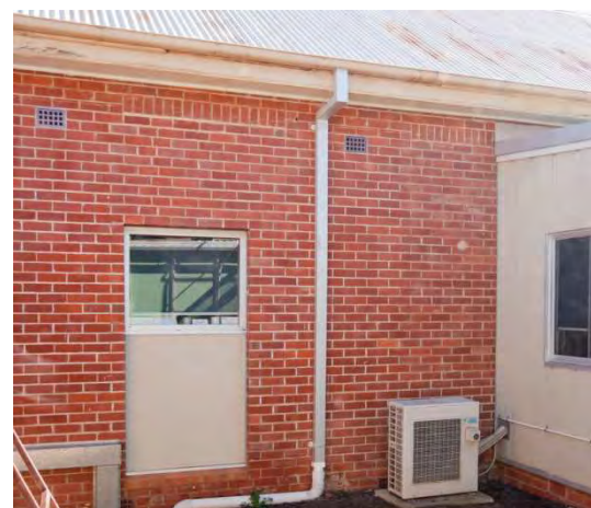
Figure 33 Lintels on east wall of 1936 f. Male Ward for the former door and window. The eaves and roof remain intact – Adaptive Architects Pty Ltd 2014
