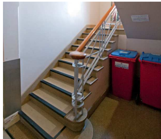
Figure 42 Original stairs are intact and add an interesting design element. Made from terrazzo treads with steel balustrades and heavy timber wreathed handrails – Adaptive Architects Pty Ltd 2014
