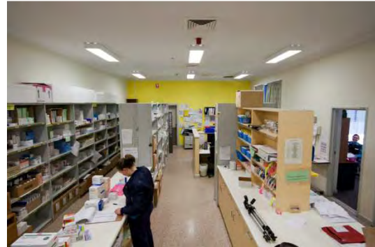
Figure 37 Internally the former Male Ward remains as a single space. The ceilings are modern, and may have been installed below original ceilings as in common in small hospitals. The internal walls have had their lime render stripped off for hard cement render. The floors are concealed and may have been concreted or are intact – Adaptive Architects Pty Ltd 2014
