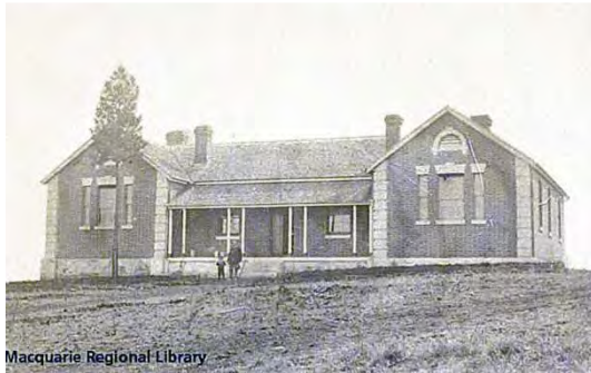
Figure 10 Alternate view of the hospital. As the tree is slightly smaller than the image above, and the site is denuded of any low planting, we can assume this is a very early shot, possibly at the building's completion 1868-1870. Macquarie Regional Library – Local Studies Collection – D0000511
