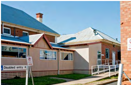
Figure 36 This view is quite instructive showing that Parkes's verandah was significantly higher than the altered verandah to the 1887 wing, and gives the dimensions to reconstruct the verandah. It also shows the surviving section of brickwork from the 1887 Fever Ward – Adaptive Architects Pty Ltd 2014
