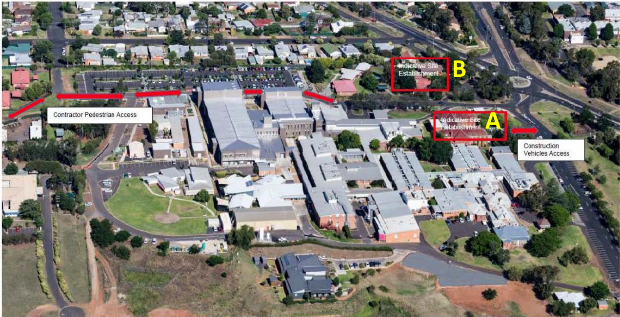
Figure 12 Proposed site establishment zones within the DHS site, compounds A and B
