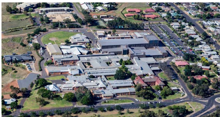
Figure 1 Aerial photo – Dubbo Hospital campus (November 2015)
