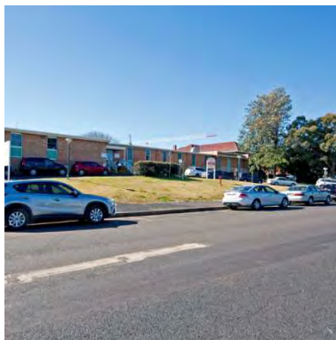
Figure 137 The 1968 building very effectively blocks the heritage streetscape to Myall Street, which is a major design element in all of the original buildings
