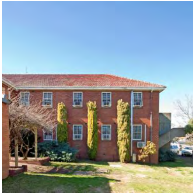
Figure 122 1936 nurses' building exterior from the west. The vertical join can be seen to the left of the third window from the end
