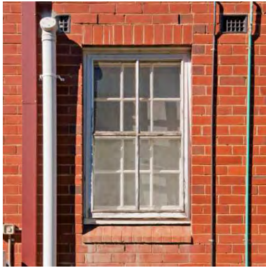
Figure 113 1936 nurses' building exterior showing typical window
