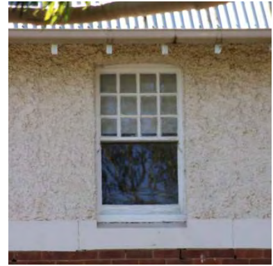
Figure 79 1907 building exterior showing feature windows
