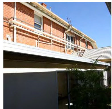
Figure 85 1907 building exterior rear showing how hospital services can impact heritage. Generally there is sensitivity in the servicing of the old building.
