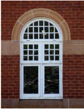
Figure 77 1907 building exterior showing feature windows
