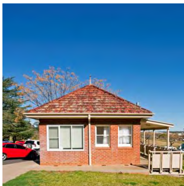
Figure 111 1936 kiosk – north elevation – the opening to the left originally had no framing
