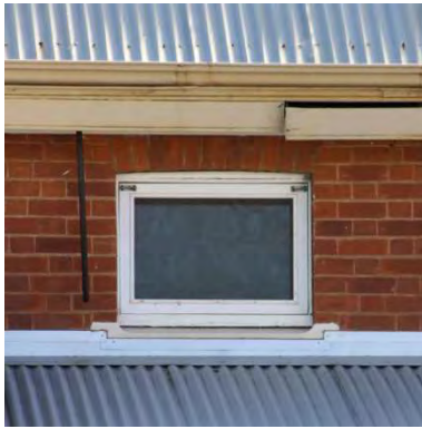
Figure 80 1887/1907 building exterior showing highlight ventilation window – note Flemish bond to brickwork
