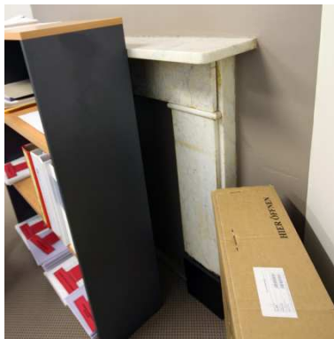
Figure 93 1907 interior upper floor showing intact original nurses' quarters – original marble fireplace
