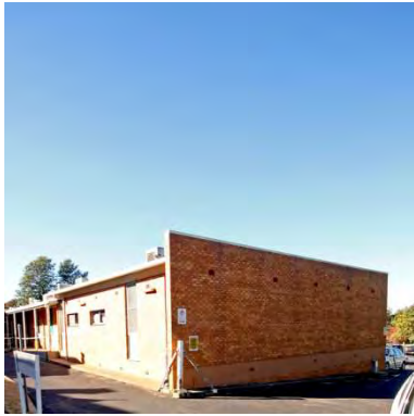
Figure 130 1968 administration building exterior from entry of 1907 building looking towards Myall Street
