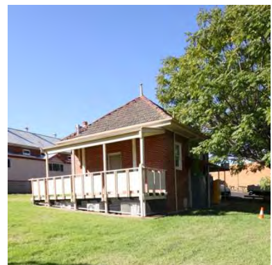
Figure 112 1936 kiosk – from south west. This building is largely intact but could be presented better
