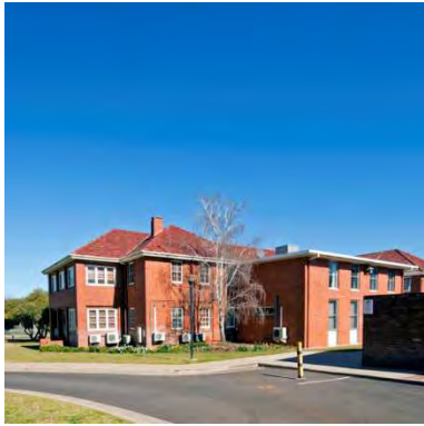
Figure 116 1936 nurses' building exterior from the north east
