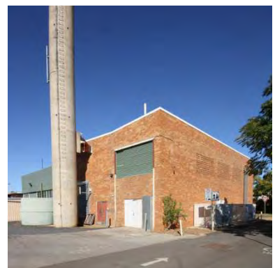
Figure 129 1962 boiler house exterior from north west – this building was demolished in the Stage 1&2 works 2012
