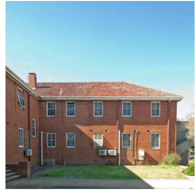
Figure 124 1936 nurses' building exterior inner court view of east bay. The vertical join is more evident on this facade, as is the impact upon the building's proportions
