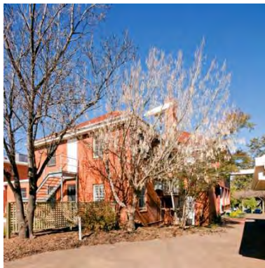
Figure 120 1936 nurses' building exterior from the north west – the chimney can be seen through the tree
