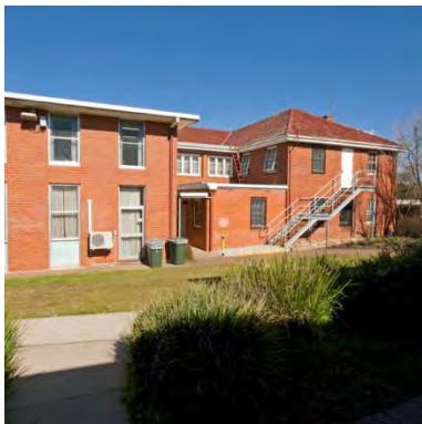
Figure 119 1936 nurses' building exterior western bay housing the conference room – later additions have greatly impacted this face
