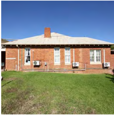
Figure 104 c1890/1926 additions exterior north face showing modifications to wall including the junction between the two
