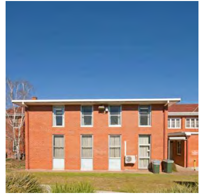
Figure 118 The c1980s addition to the 1936 nurses' building – this addition blocks the long northern open verandahs on the original building
