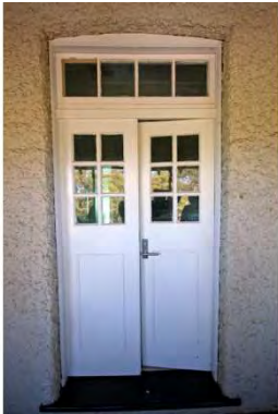
Figure 95 1907 exterior upper floor showing balcony doors
