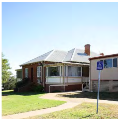
Figure 102 1926 additions to 1868 building exterior showing change to hipped roof
