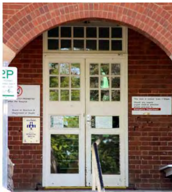
Figure 74 1907 building exterior showing intact main entry door inside brick arch
