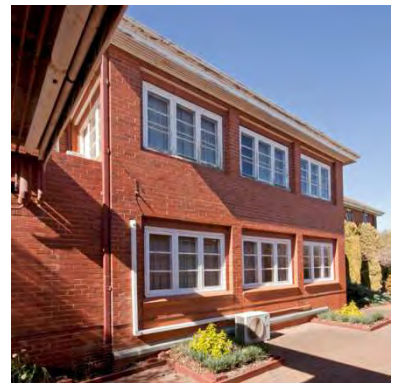
Figure 121 1936 nurses' building exterior western balcony, also infilled with later windows
