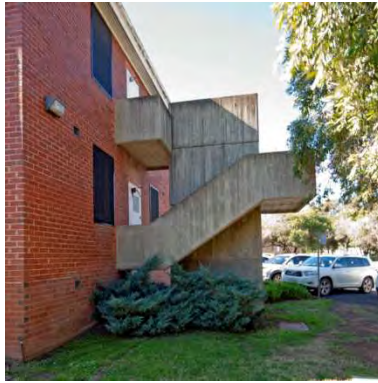
Figure 123 1936 nurses' building fire stairs
