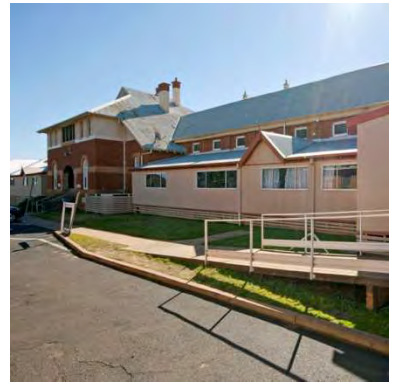
Figure 135 View of the heritage block from the south east is one of the better views, completely blocked by the 1968 administration building
