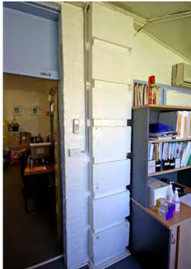
Figure 61 1868 building exterior corner showing original pilaster
