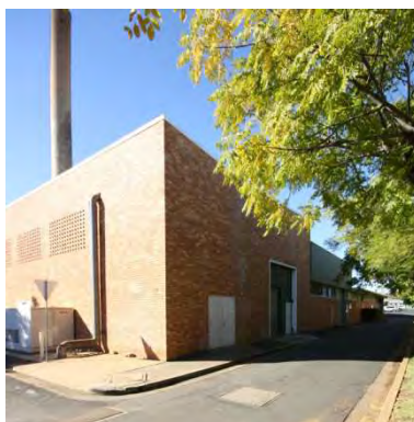
Figure 128 1962 boiler house exterior from south west – this building was demolished in the Stage 1&2 works 2012
