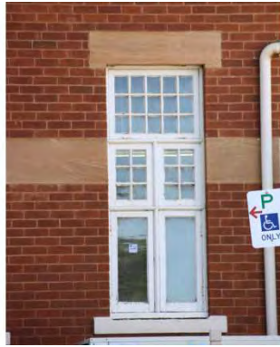
Figure 78 1907 building exterior showing feature windows
