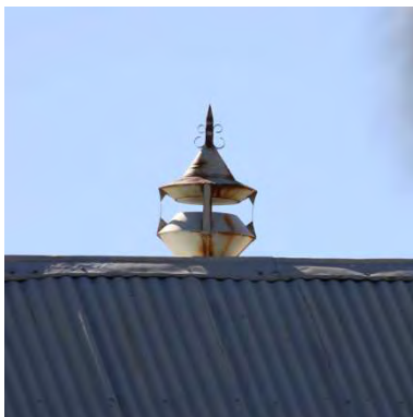
Figure 83 1907 building exterior showing roof ventilator
