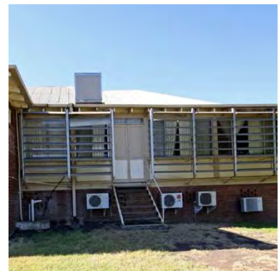
Figure 103 1926 additions to 1868 building exterior showing verandah. The c1970 louvres have not survived well and are now detracting from the building
