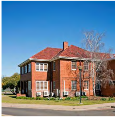
Figure 117 1936 nurses' building exterior Showing the intact eastern bay and transverse balcony with openings infilled by later windows
