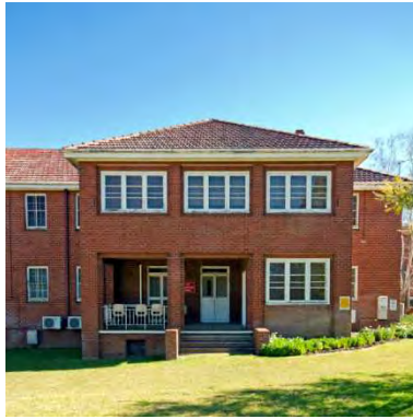
Figure 126 1936 nurses' building east view of balcony with later infilled windows
