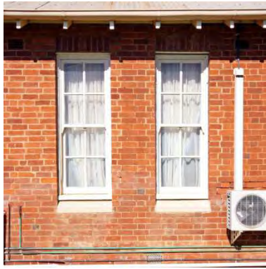
Figure 105 c1890 additions exterior north face showing 1926 windows cut into wall. The discoloured mortar shows where bricks were removed. Wells' drawings show these as 12 pane d/h
