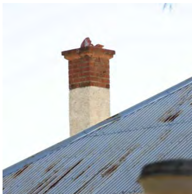
Figure 84 1907 building exterior showing original chimney
