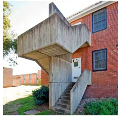
Figure 115 1936 nurses' building exterior showing later fire stairs
