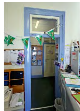
Figure 69 c1890 additions to 1868 building interior showing early intact doorset. All other architraves were stripped out 1926
