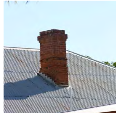
Figure 63 1868 building exterior showing original chimney
