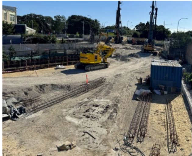
Picture 2 North-eastern corner of site on Syd Einfeld Drive
