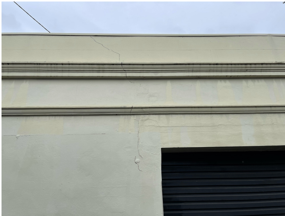
Photo 3 Cracking of garage wall
