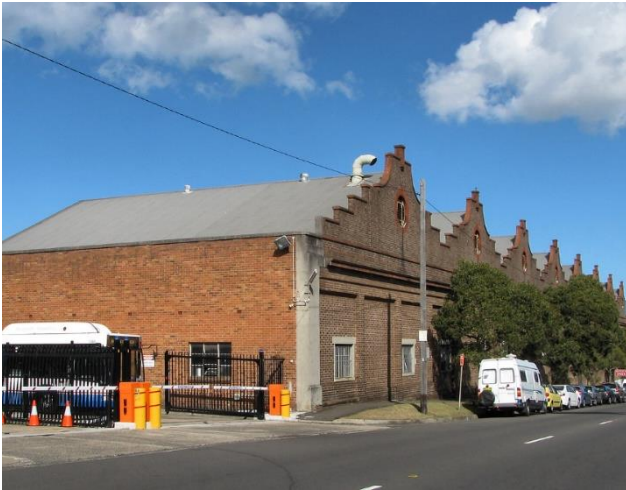
Picture 11 Waverley Tram Depot Building, I224
