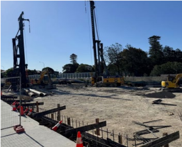
Picture 1 Site from York Road, off Syd Einfeld Drive Source: SJB
