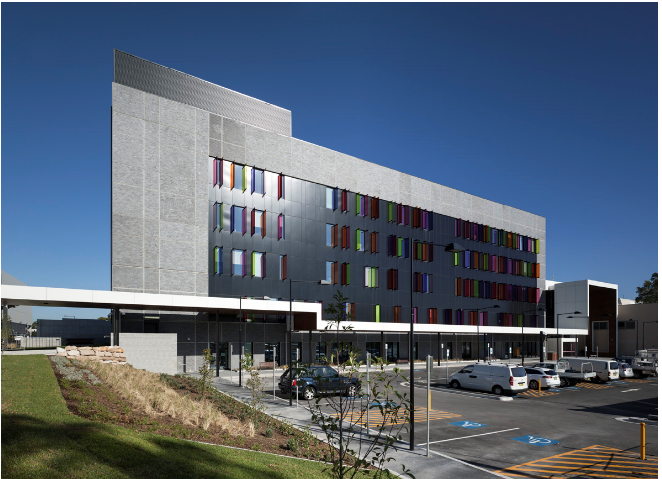
Stage 1 CSB east facade
