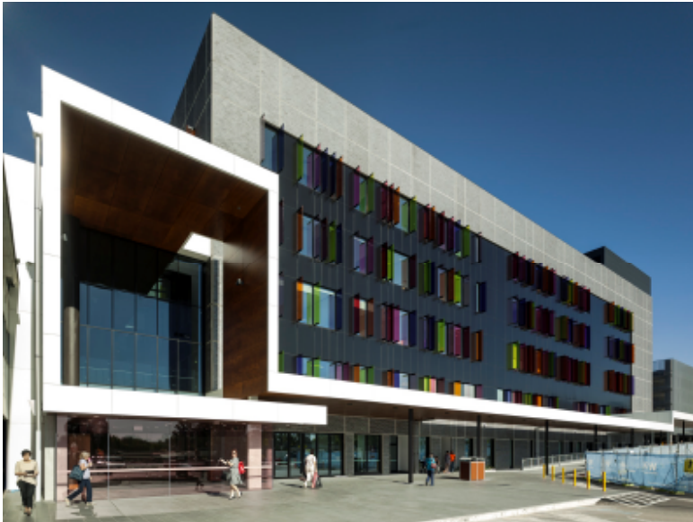
Stage 1 CSB west façade
