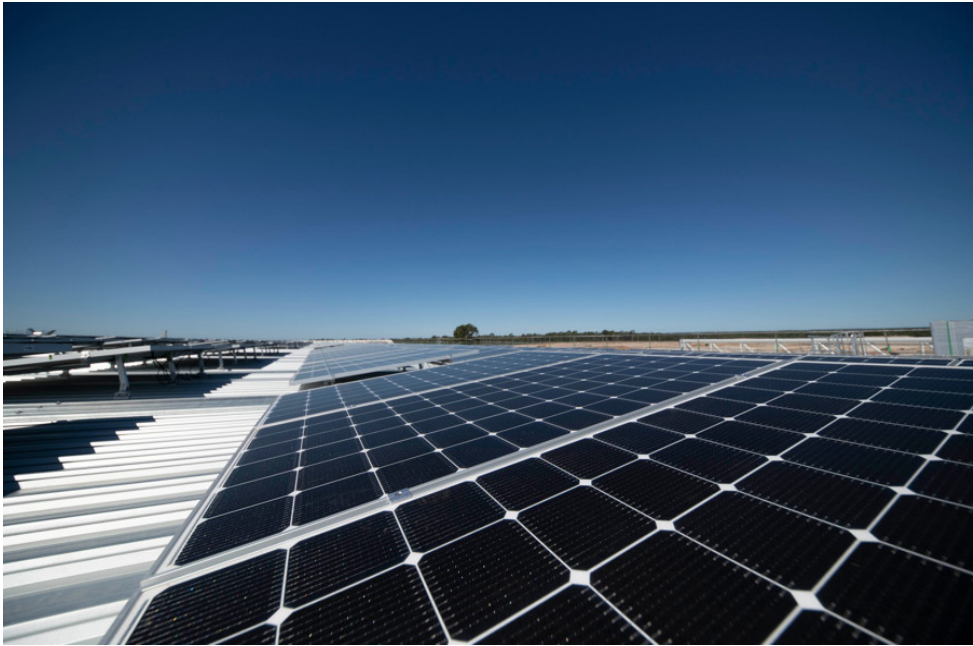
FIGURE 2.8 - Solar Panels installed at development East Warehouse 1. Alone, this installation generates 4,800MWh per year, or the equivalent of powering more than 7,300 homes.
