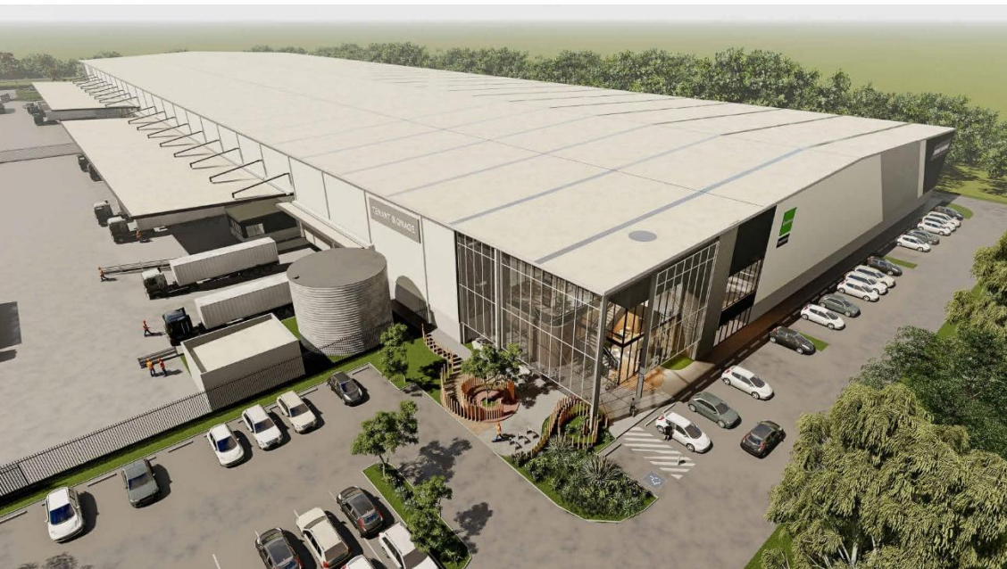
Figure 13: Aerial view from south-west of Warehouse 2B-2 (Source: SBA Architects)
