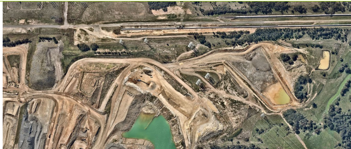
Photo 21. Aerial photograph (October 2020)
