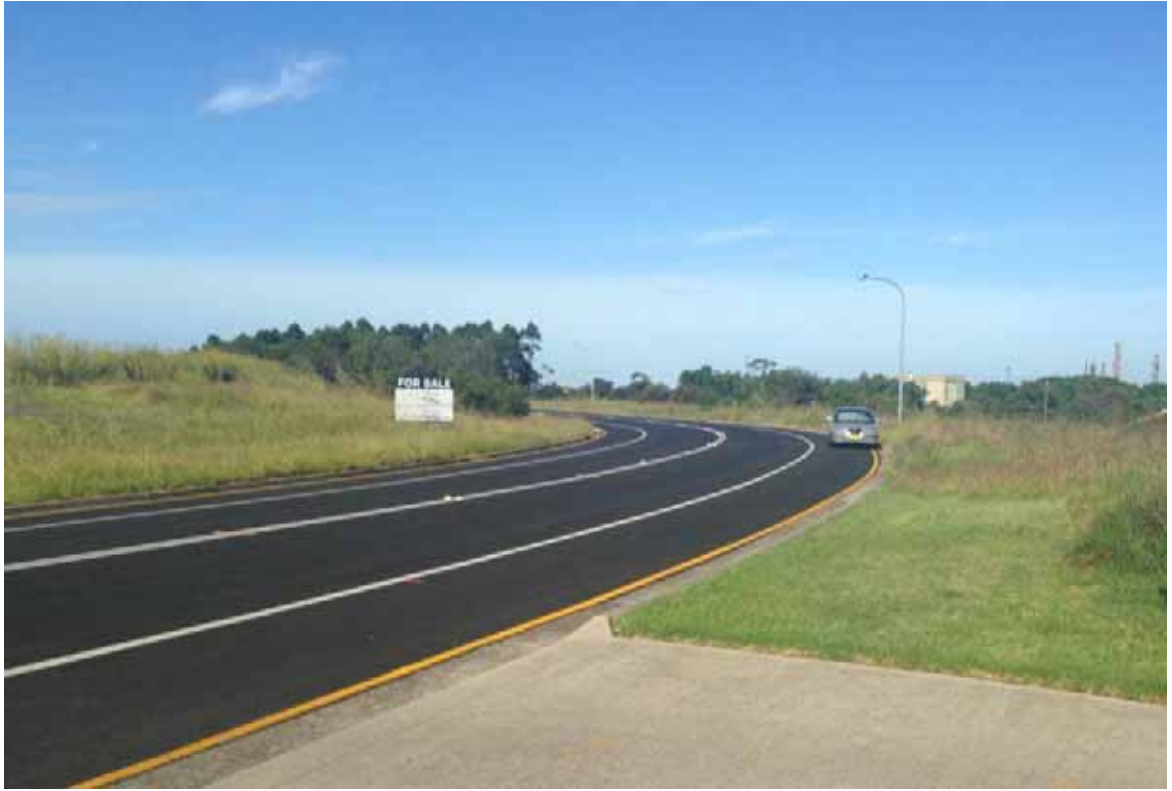
Photograph 2.4 Murray Dwyer Circuit at the corner 300 metres south of the site
