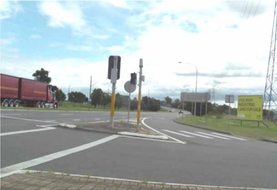
Photograph 2.6 Industrial Drive looking west from Steel River Boulevard
