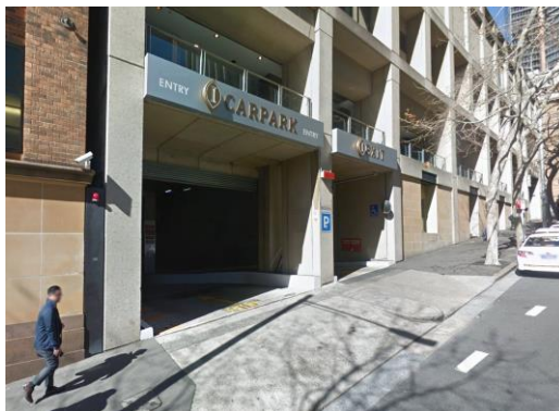
Car park entry
