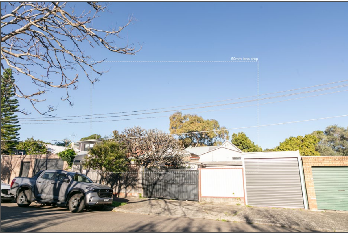
ORIGINAL PHOTOGRAPH SHOWING CURRENT CONDITION
