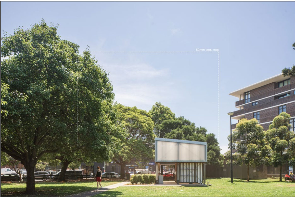
ORIGINAL PHOTOGRAPH SHOWING CURRENT CONDITION
