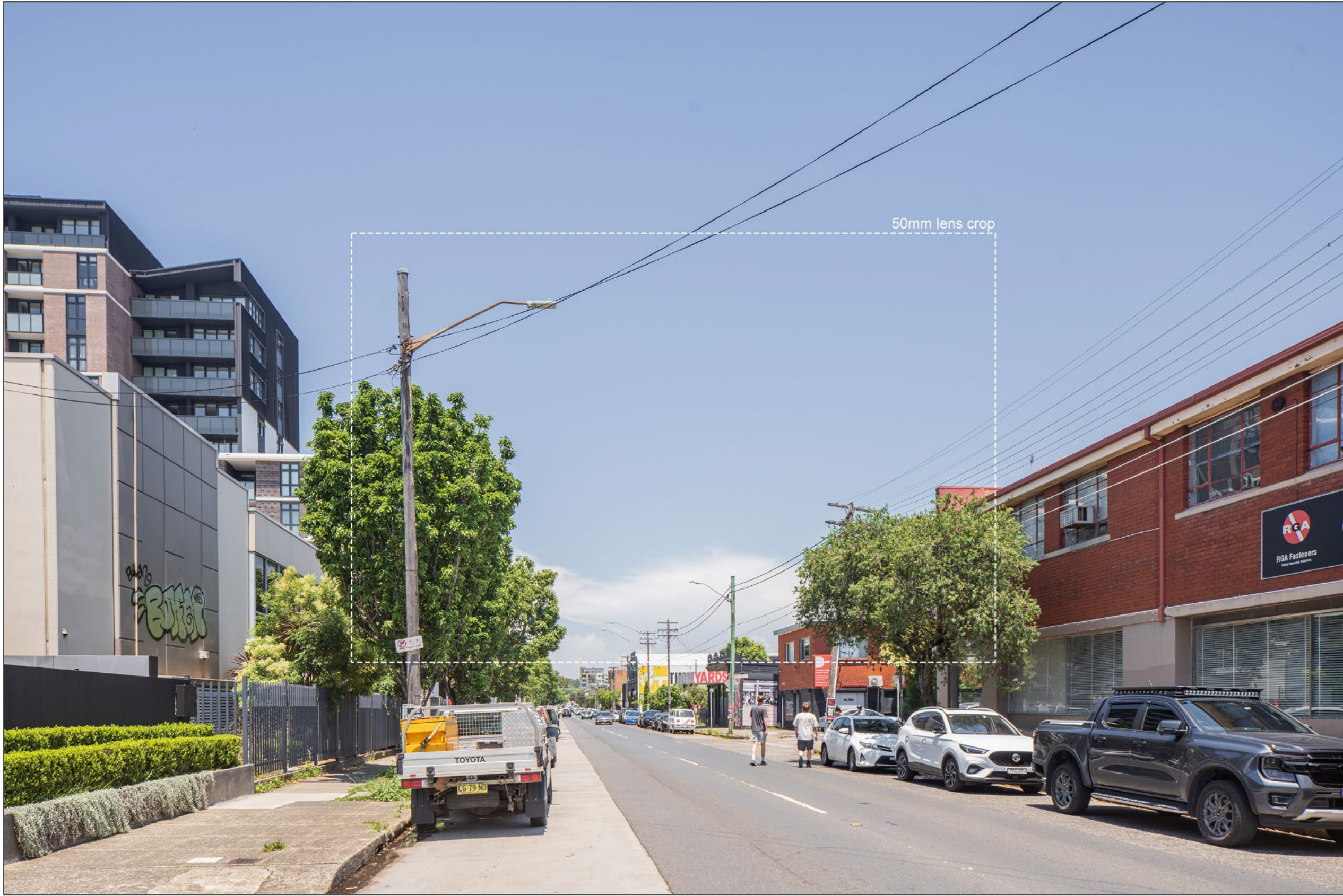
ORIGINAL PHOTOGRAPH SHOWING CURRENT CONDITION
