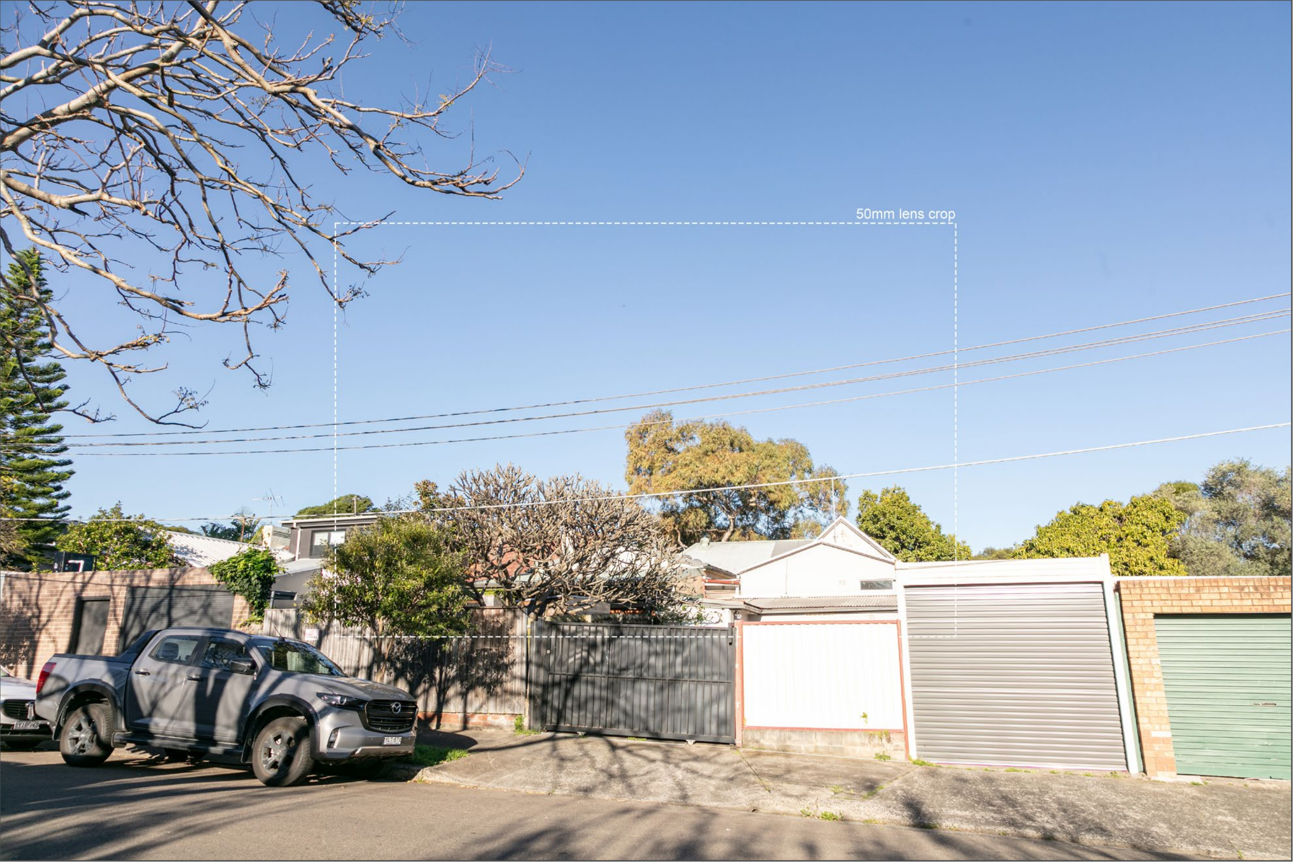
ORIGINAL PHOTOGRAPH SHOWING CURRENT CONDITION
