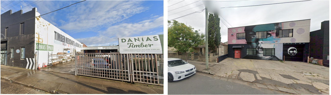
Figure 8 Existing site conditions (Timberyards on left and warehousing adjacent dwellings on right)
