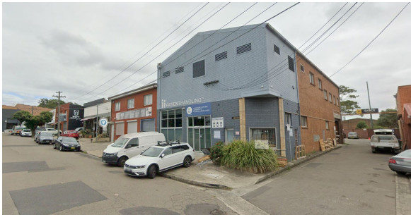
Northeast: Street view of Mitchell Street
