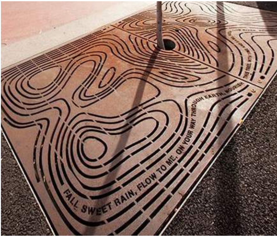
Figure.38 - Image | Tree pit with water collection structure
