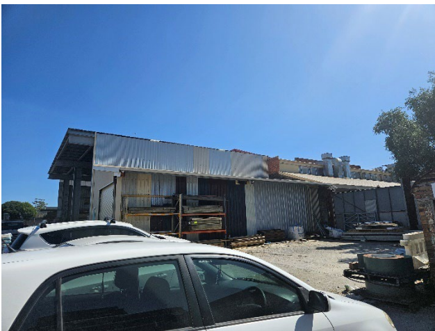
figure 32 View looking south west from within the timber yard, (183 Victoria Road).
