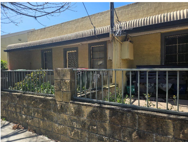
Figure 70 Part of the group of cottages situated on Farr Street.
