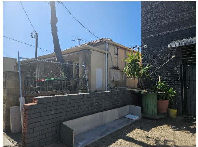
Figure 55 Factory building located at 135 Sydenham Road, with partial view of dwelling at 7 Farr Street.
