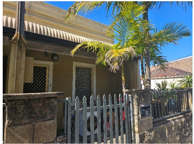
Figure 63 Part of the group of cottages situated on Farr Street.
