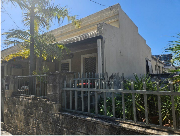
Figure 60. Part of the group of cottages situated on Farr Street.
