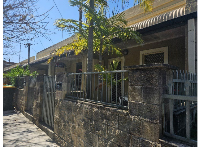
Figure 61 Part of the group of cottages situated on Farr Street.
