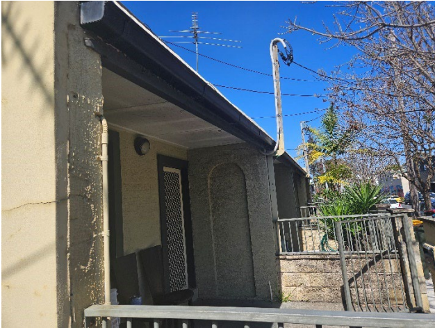
Figure 66 Part of the group of cottages situated on Farr Street.
