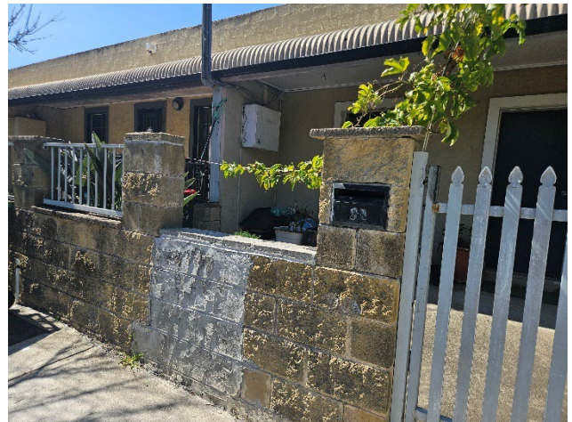
Figure 69 Part of the group of cottages situated on Farr Street.
