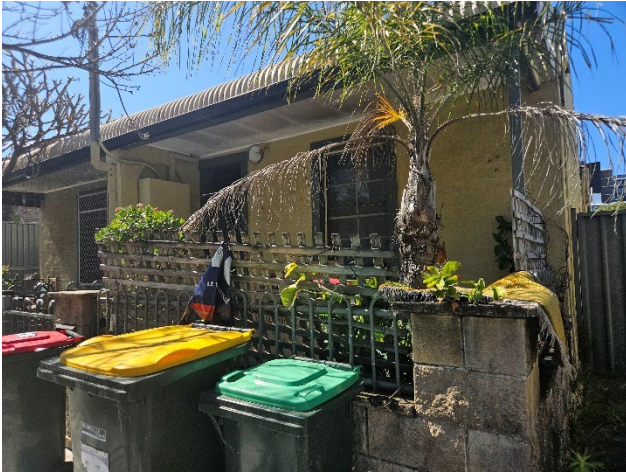
Figure 72 Part of the group of cottages situated on Farr Street.
