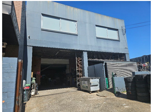
Figure 19 Building located at 4 Mitchell Street.
