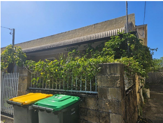
Figure 68 Part of the group of cottages situated on Farr Street.
