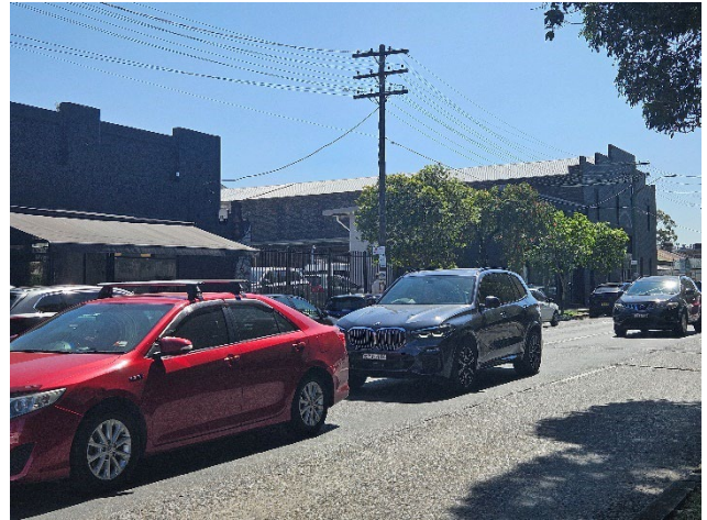
Figure 39 View looking north east along Victoria Road.
