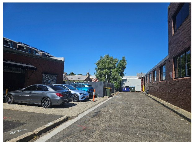
Figure 15 View looking south west along lane way located on Mitchell Street.
