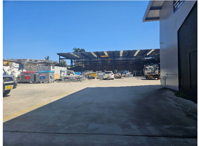
Figure 37 View looking south west outside large factory located within the timber yard (183 Victoria Road).
