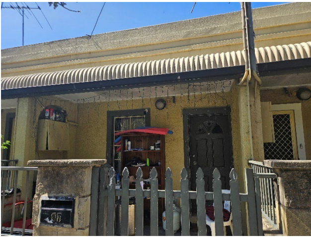
Figure 62 Part of the group of cottages situated on Farr Street.
