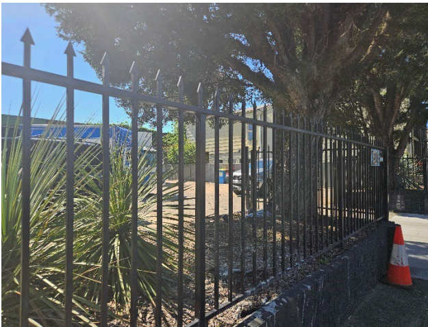
Figure 42 View looking at gated area of 119A – 121 Sydenham Road.
