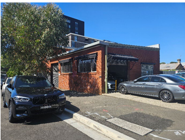
Figure 14 View looking south at building located at the corner of Victoria Road and Mitchell Street (165 Victoria Road).
