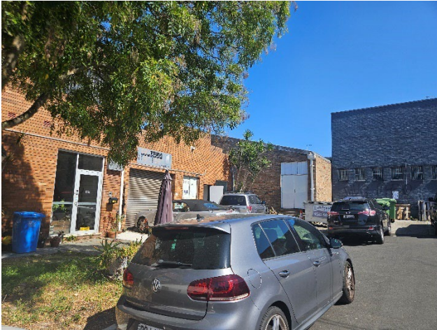
Figure 22 Building located at 1/10-14 Mitchell Street, showing part of building located at 35 Farr Street.
