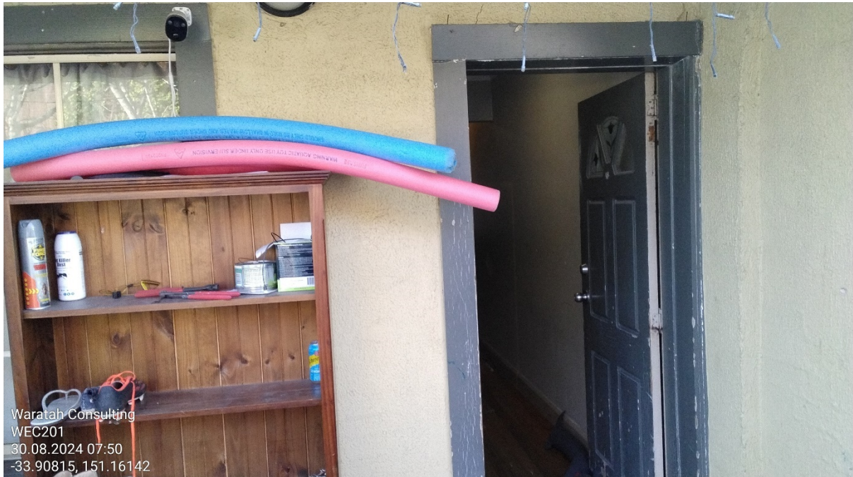
Photograph 9: 17 Farr Street, exterior (30/08/24)
