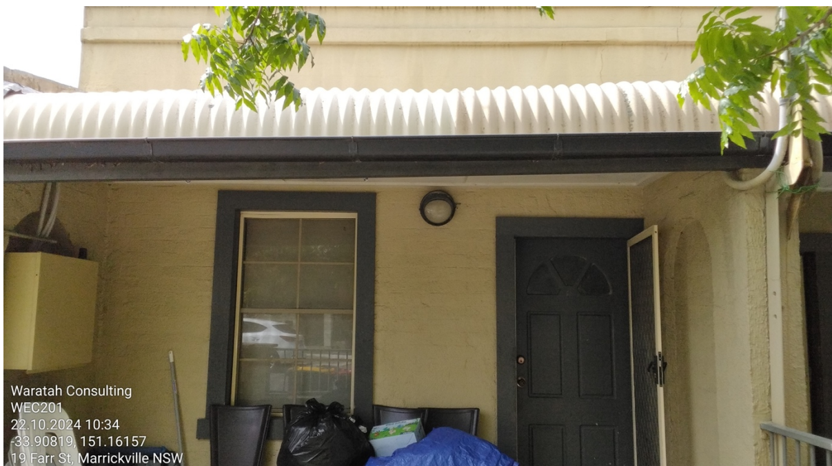
Photograph 40: 21 Farr Street, exterior, walls, render, yellow paint system (22.10.24)
