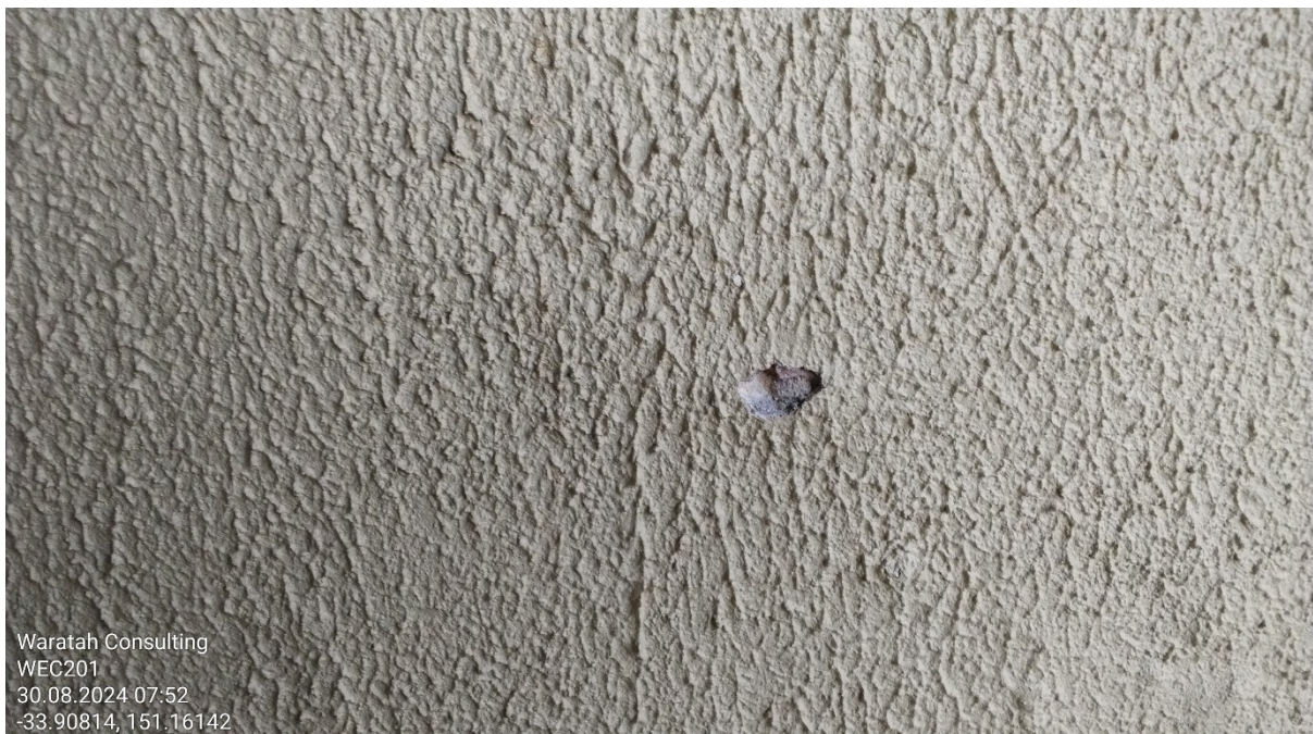
Photograph 10: 17 Farr Street, exterior, walls, render throughout, yellow paint system Pb201 (30/08/24)
