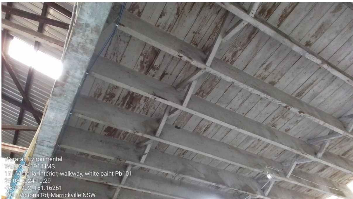
Photograph 2: 191 Victoria, interior, underside of walkway, white paint system (28/08/24)
