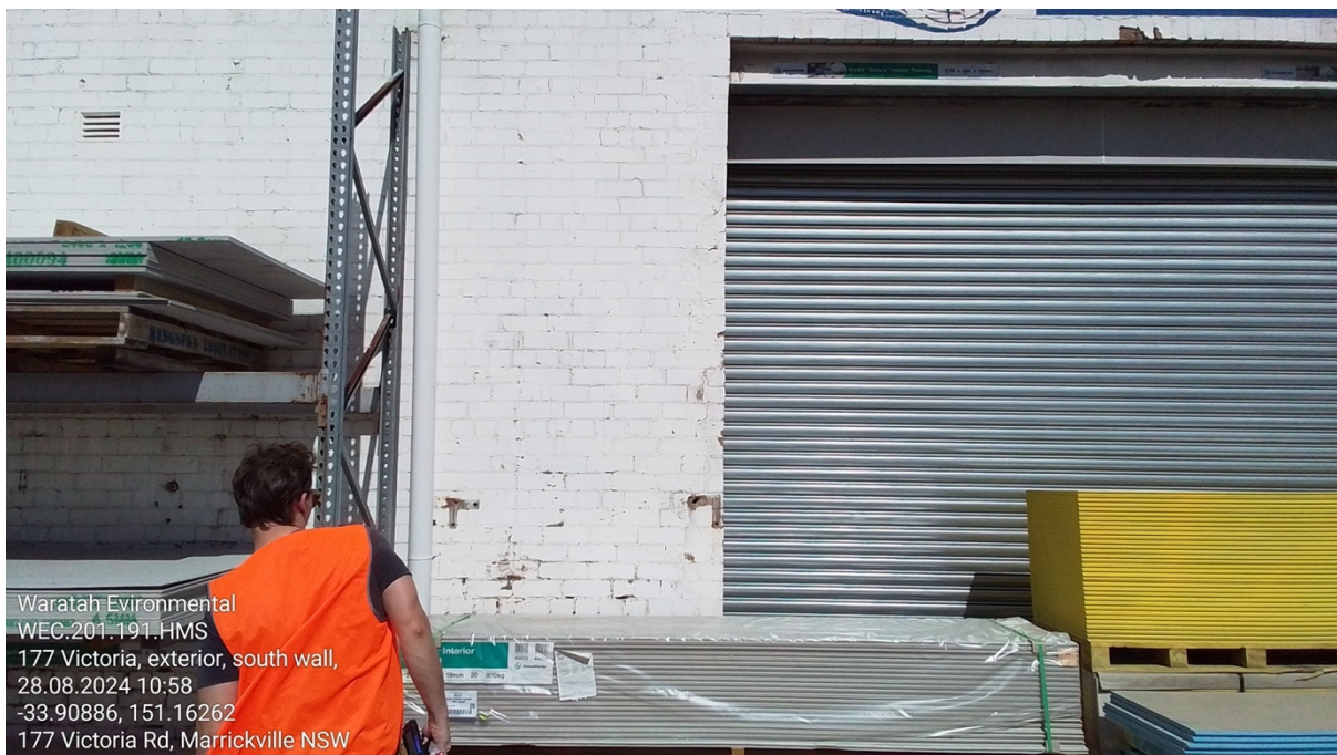
Photograph 8: 177 Victoria, exterior, south wall, white paint system (28/08/24)
