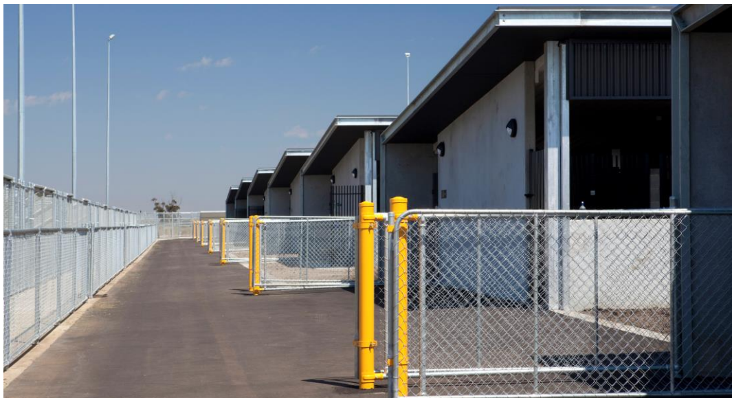
Figure 15 – Melbourne Customs Facility
