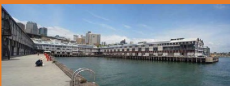
Wharf 4/5 viewed from Pier 2/3 western apron
