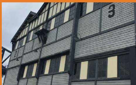
Pier 2/3 northern elevation
