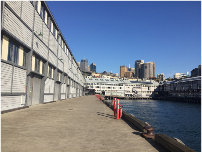
Figure 25 West apron Pier 2/3
