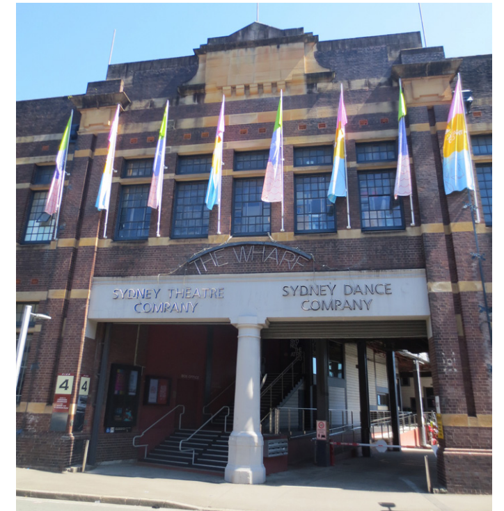
Figure 7 Hickson Road entry to Wharf 4/5
