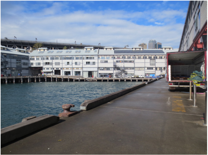
Figure 24 East apron Wharf 4/5
