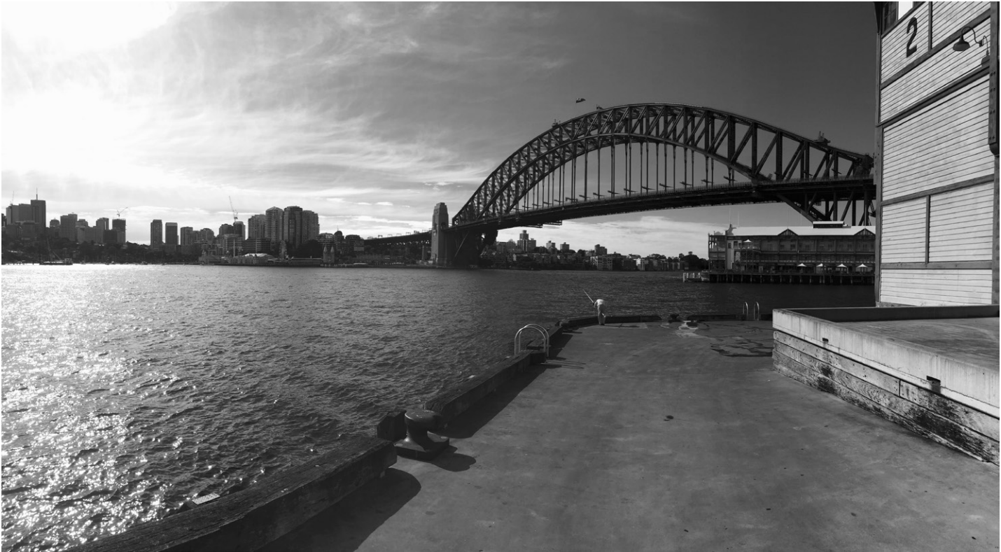
Figure 23 North apron Pier 2/3
