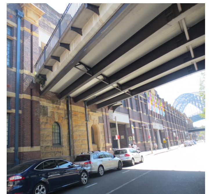
Figure 8 Hickson Road view towards Harbour Bridge
