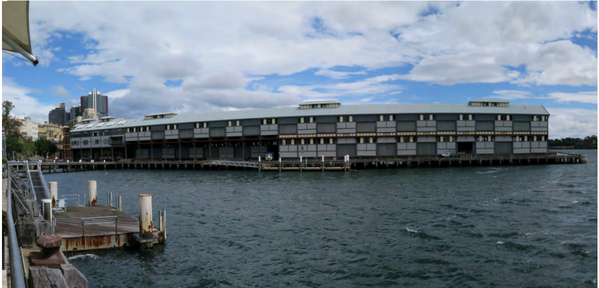
Figure 16 Eastern side of Pier 2/3. (Source: CRM 2016)
