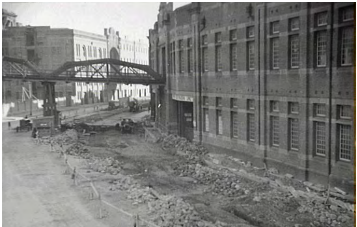
Figure 14 Looking southwest along Hickson Road opposite Walsh Bay Wharves 6-9, circa 1933 (Source: City of Sydney Archives SRC6609)
