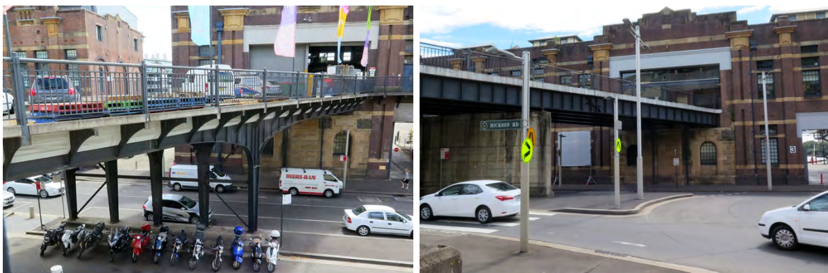
Figure 22 Bridges from Pottinger Street to Wharf 4/5 (L) and Pier 2/3 (R). (Source: CRM 2016)
