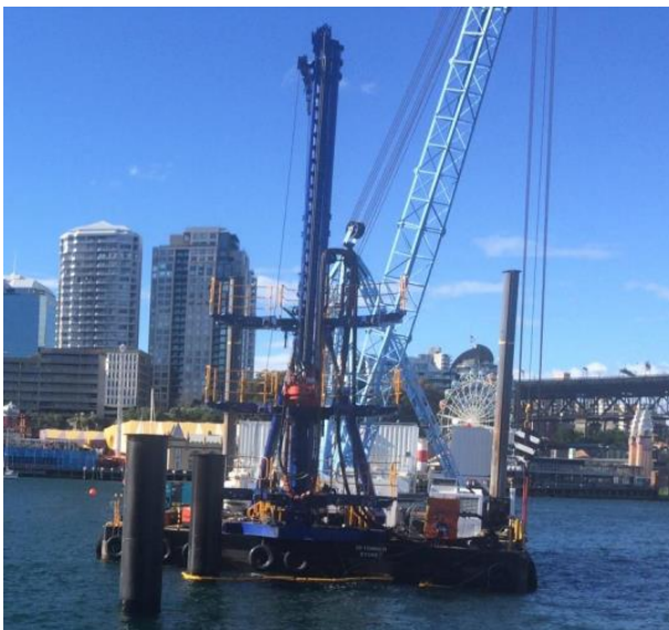
Figure 13: Piling rig used for inserting screwed piles
