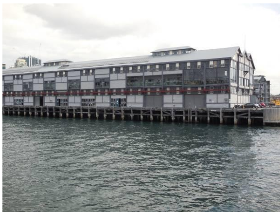
Figure 27: Wharf 4/5 East elevation
