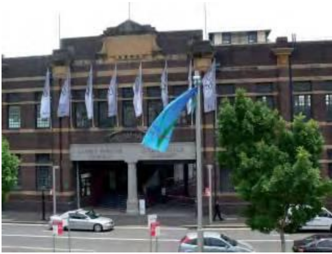
Figure 37: Shore Sheds South elevation
