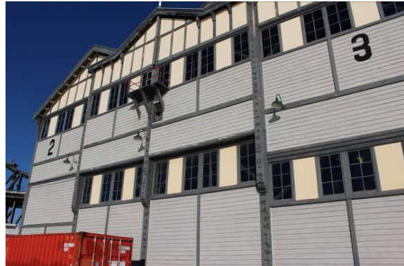
Figure 14: Pier 2/3 North elevation
