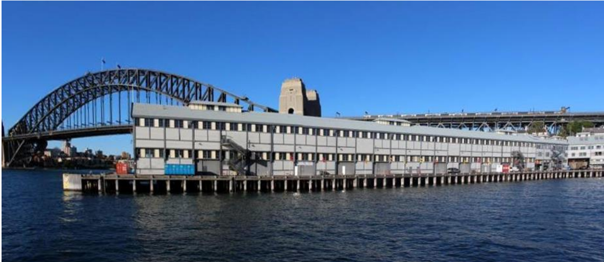
Figure 12: Pier 2/3 West elevation
