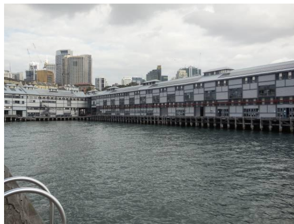
Figure 28: Wharf 4/5 East elevation
