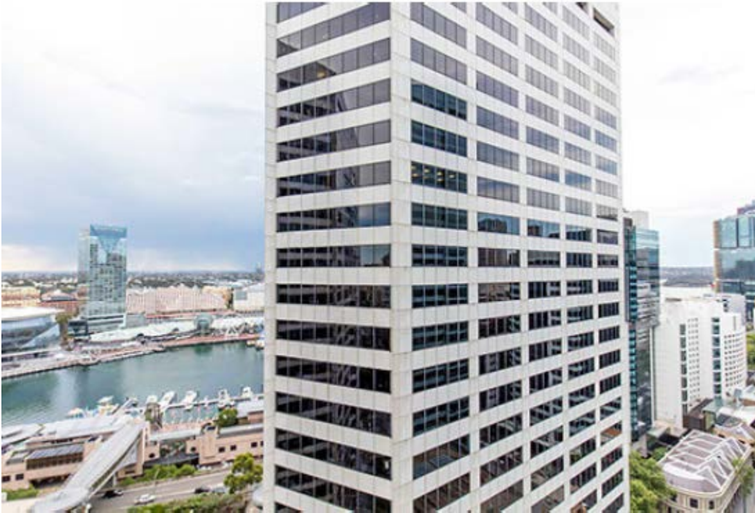
Figure 103 Oblique view to the north west from Apartment 100
