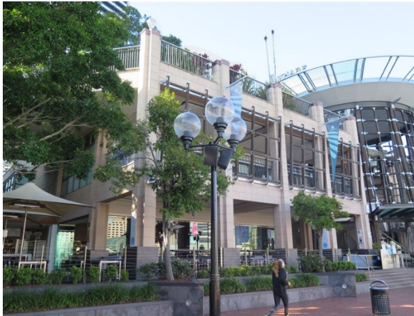
Figure 3.9 Looking southeast at the northern end of the existing Cockle Bay Wharf. (Source: GML, 2016)
