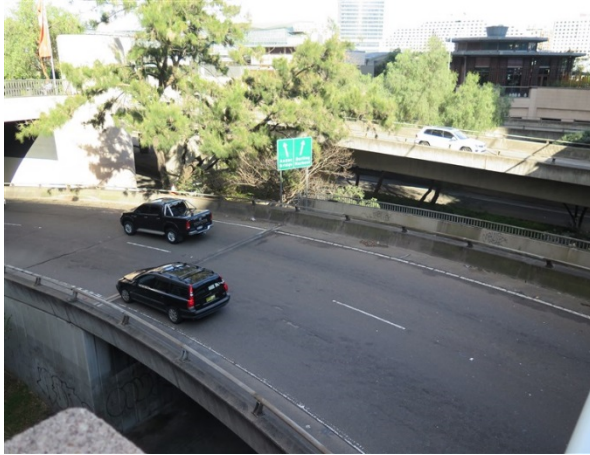
Figure 3.15 Looking southwest across the Western Distributor flyovers located in the northern part of the study area. Cockle Bay Wharf is visible in the background of the image (Source: GML, 2016)
