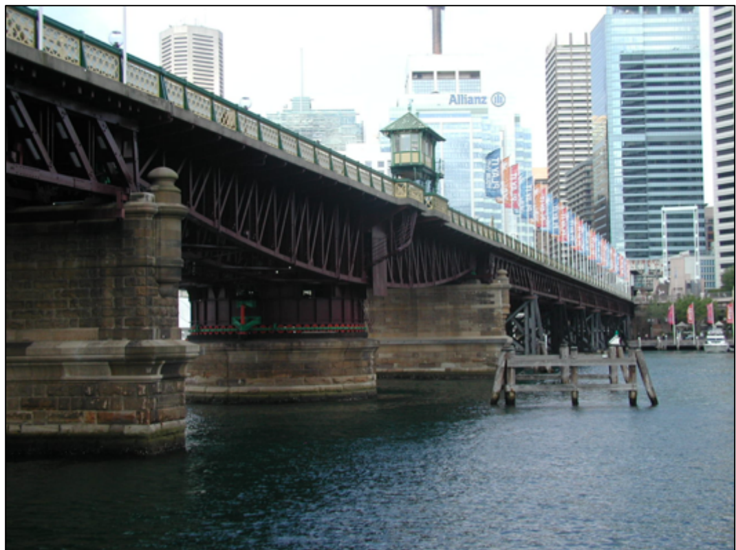
Figure 12: Pymont Bridge looking towards the development site. West Sydney Harbour Ferry Tour
