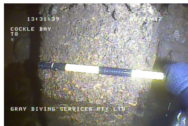
Figure 88: Close up of sheet piling. Scale is in 100 mm increments. (Cockle Bay 170821 T8, 7:07)
