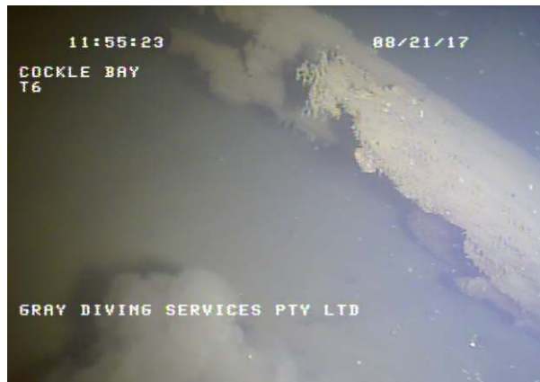
Figure 72: Single timber pile protruding north-east. (Cockle Bay 170821 T6, 3:06)
