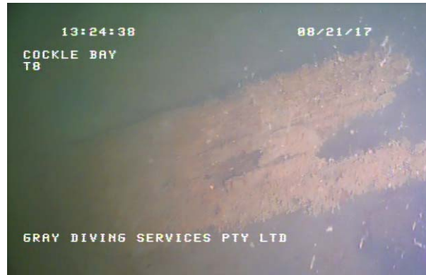
Figure 84: Timber pile on Transect 8. (Cockle Bay 170821 T8, 0:40)
