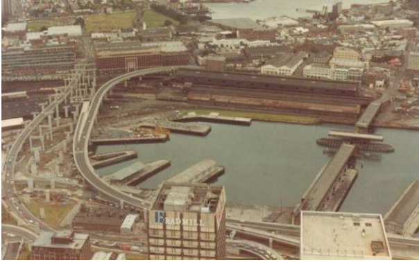
Figure 31: 1984 aerial photograph showing early stages of demolition of railway yards and wharves. 46
