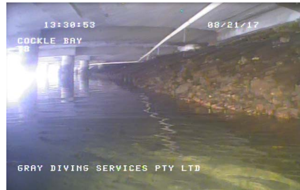
Figure 86: Looking north along seawall with rock embankment spilling over sheet piling, but the sheet piling becoming visible again approximately two piers down. (Cockle Bay 170821 T8, 6:25)
