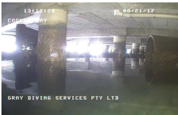
Figure 82: Timber diffuser or barrier in front of the storm water outlet, behind the D steel pier. (Cockle Bay 170821 T7, 4:53)
