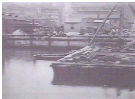
Figure 44: Completed Monier plate facing of seawall between Wharves 35 and 36, Darling Harbour, 1919. 55
