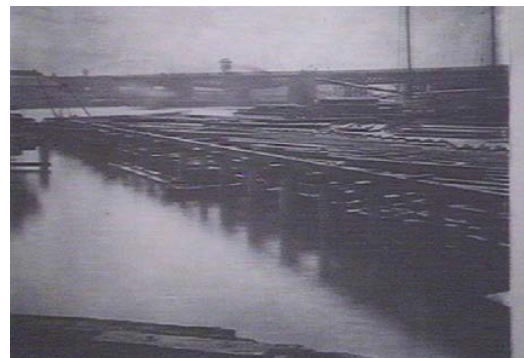
Figure 23: Wharf 35 under construction, September 1918. 38
