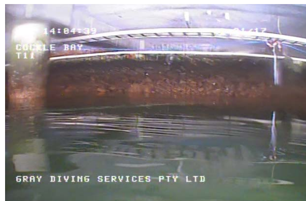
Figure 98: Second rock embankment against the seawall at the C steel piers. (Cockle Bay 170821 T11, 4:35)
