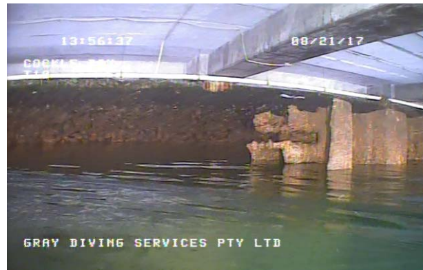
Figure 94: Visible end of sheet piling above water, with shadow of continued sheet piling below water level. Rock embankment and concrete seawall in background around the C steel pier. (Cockle Bay 170821 T10, 4:34)
