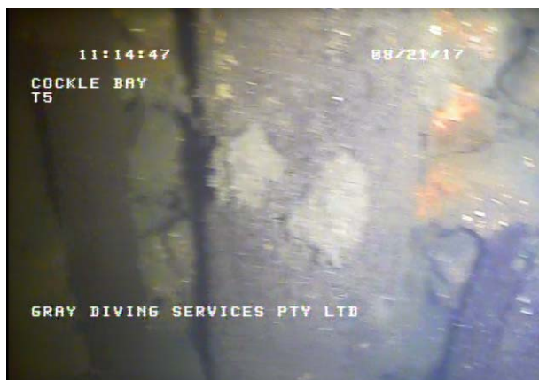
Figure 66: Northern group of three timber piles. (Cockle Bay 170821 T5, 6:27)
