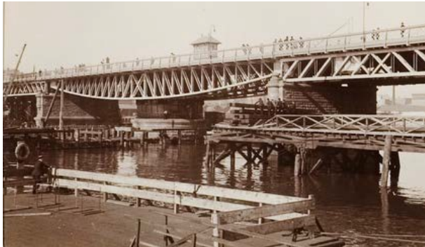
Figure 16: Pyrmont Bridge just after completion, with remnants of original bridge in foreground, 1902. 31
