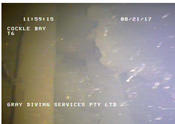
Figure 77: Some of the piles in group to the south with piece of possible concrete plating. (Cockle Bay 170821 T6, 6:40)
