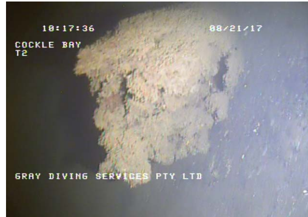
Figure 57: Timber pile protruding from rock embankment at 30 m from edge of wharf. (Cockle Bay 170821 T2, 5:55)
