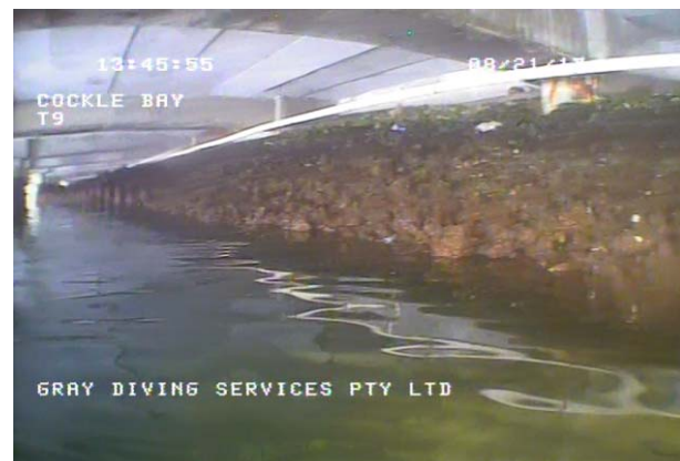
Figure 91: Seawall with rock embankment, looking north to where the sheet piling continues. (Cockle Bay 170821 T9, 3:11)
