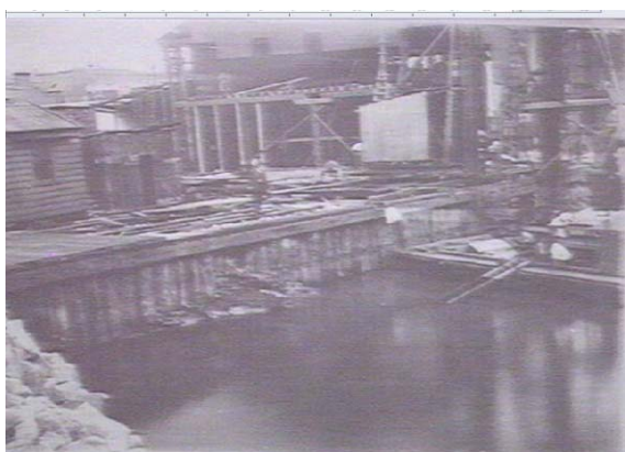
Figure 43: Timber sheet piling between Wharves 35 and 36, Darling Harbour, 1919. 54
