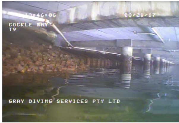
Figure 92: Seawall with rock embankment, looking south to where the sheet piling continues. (Cockle Bay 170821 T9, 3:20)
