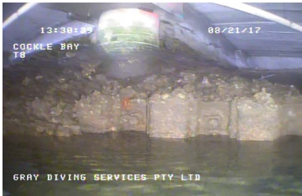
Figure 85: Sheet piling at the end of Transect 8, in front of the D steel pier with more rock embankment behind. (Cockle Bay 170821 T8, 6:12)
