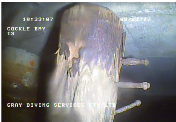
Figure 60: Top of the timber pile forming part of the diffuser. (Cockle Bay 170821 T3, 5:59)
