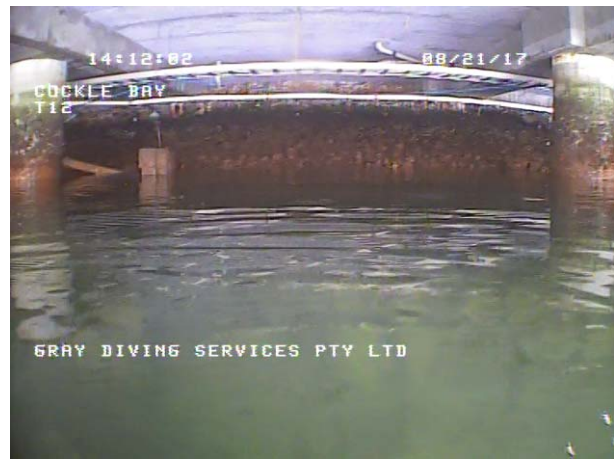
Figure 102: Second rock embankment with end of sheet piling above the water level to left, to the inside of the C pier. (Cockle Bay 170821 T12, 4:33)
