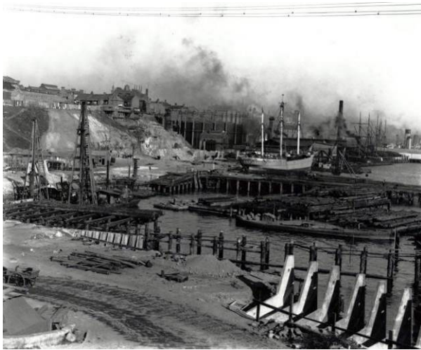
Figure 39: Example of Monier trestle seawall being constructed, Darling Harbour, 1909. 51
