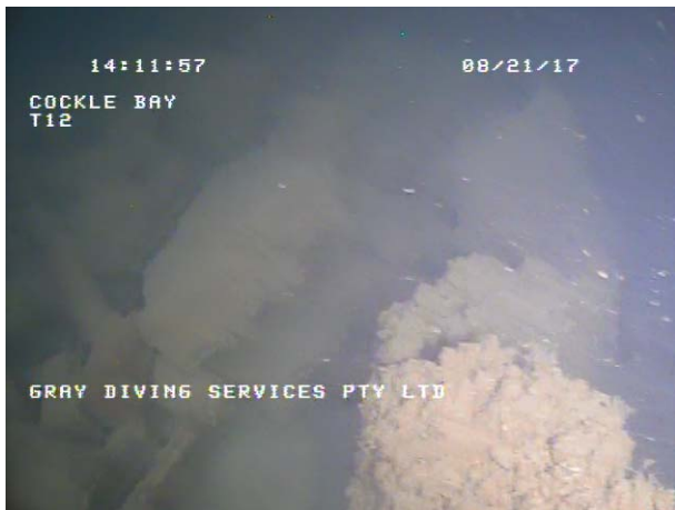
Figure 101: Corner of the sheet piling where it turns east, with debris. (Cockle Bay 170821 T12, 4:28)
