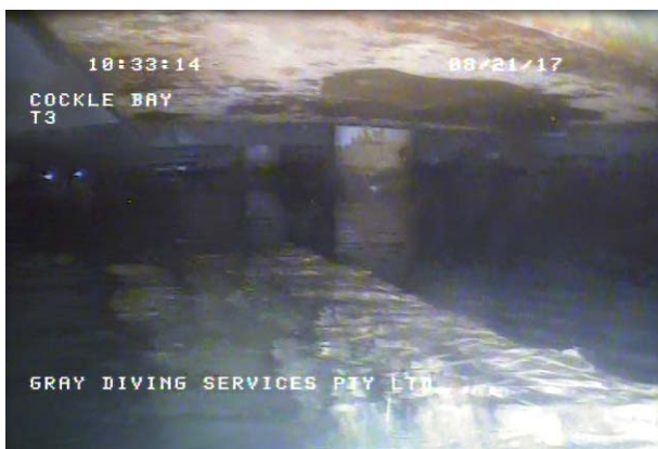
Figure 62: View north along the top of the diffuser, showing other steel piers in background. (Cockle Bay 170821 T3, 6:04)
