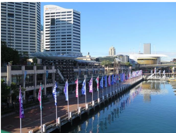
Figure 3.4 Looking southeast towards the site from Pymont Bridge. (Source: GML, 2016)
