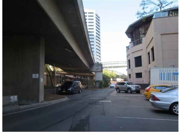
Figure 3.13 Looking south along Wheat Road in the northern part of the site. Cockle Bay Wharf is visible on the right and the Western Distributor northbound flyover is on the left. (Source: GML, 2016)
