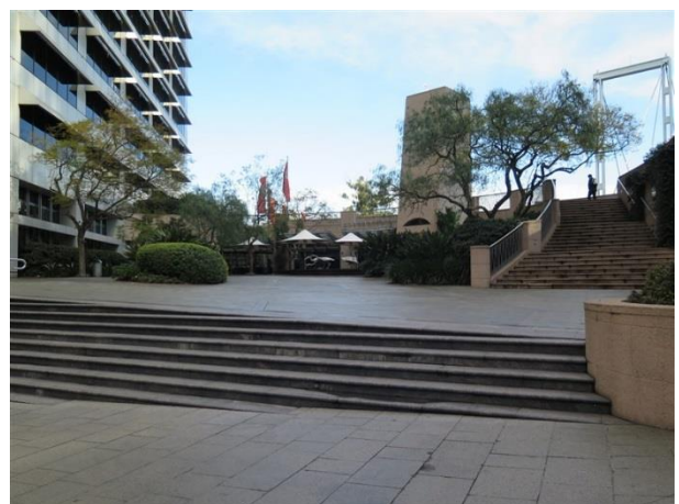
Figure 3.11 Looking west across the public domain space in the northeast of the site. (Source: GML, 2016)
