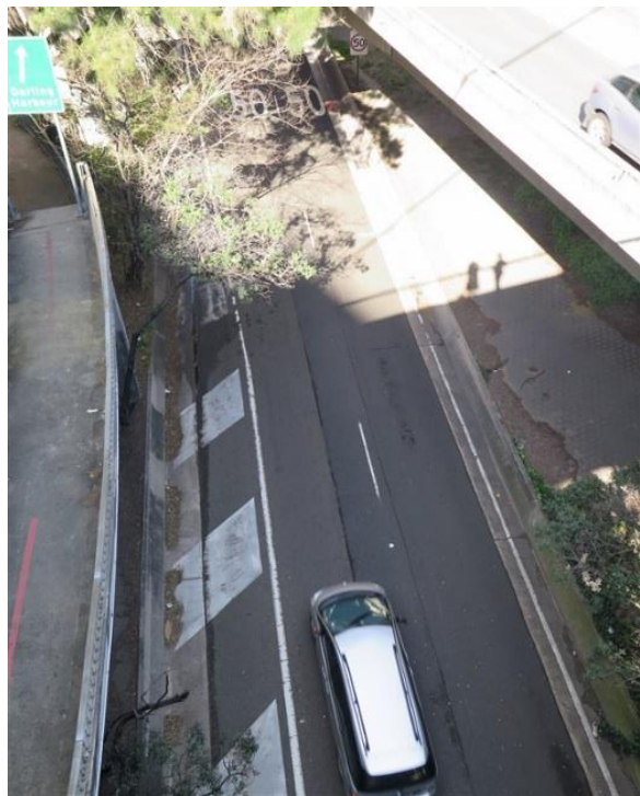
Figure 3.15 Looking down on the Western Distributor southbound lane from the pedestrian footbridge on the northern edge of the site. The northbound flyover is visible in the top right corner of the image. (Source: GML, 2016)
