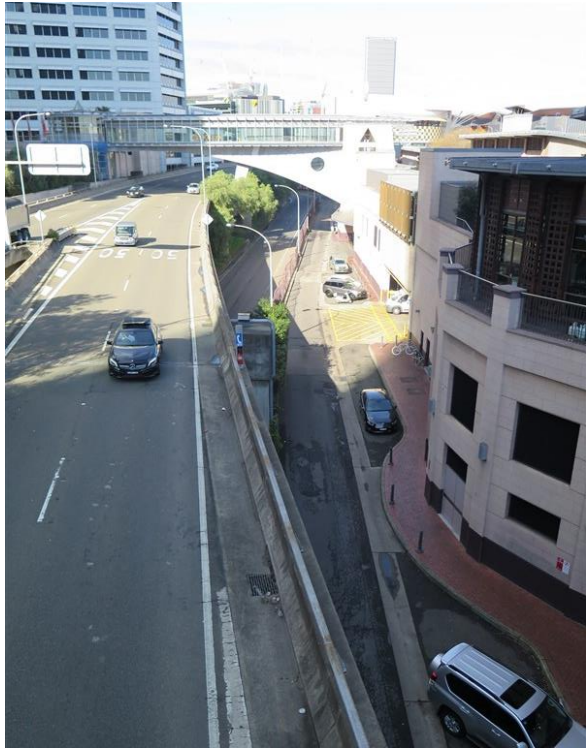
Figure 3.16 Looking south across the Western Distributor northbound flyover lane, Wheat Road, and the eastern façade of Cockle Bay Wharf from the pedestrian footbridge on the northern edge of the site. (Source: GML, 2016)
