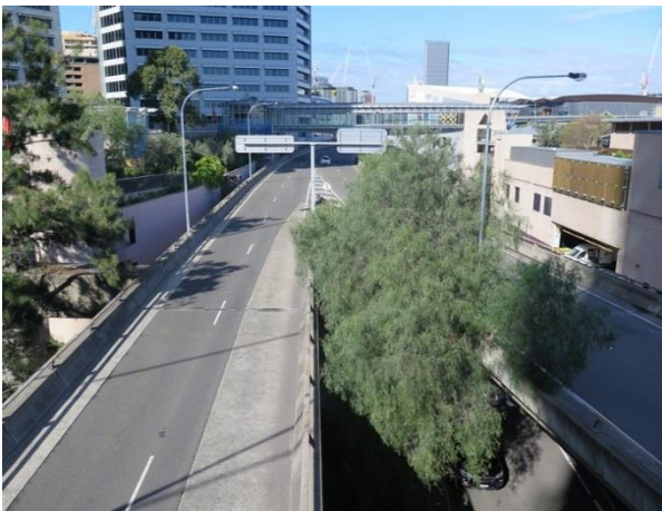
Figure 3.14 Looking south across the Western Distributor northbound flyover lanes in the northern part of the site. (Source: GML, 2016)
