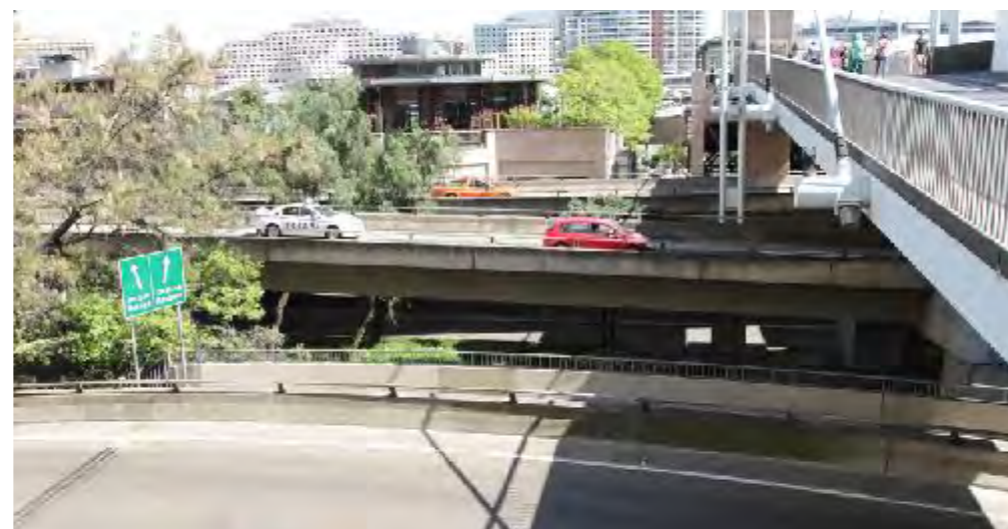
Fig. 9. Photos of existing pedestrian bridge over the Western Distributor showing the unpleasant pedestrian experience generated by heavy traffic.
